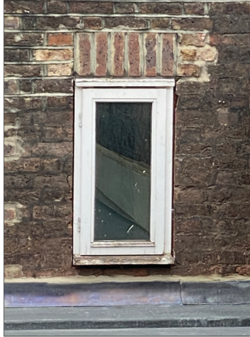
Window Detailing to match existing adjacent window
