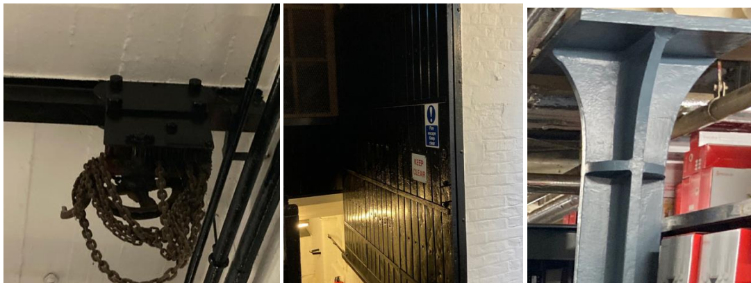
Figure 2.3: Existing historic industrial details including steel gantry crane (left), historic timber sliding doors (centre), and cast iron columns (right)
