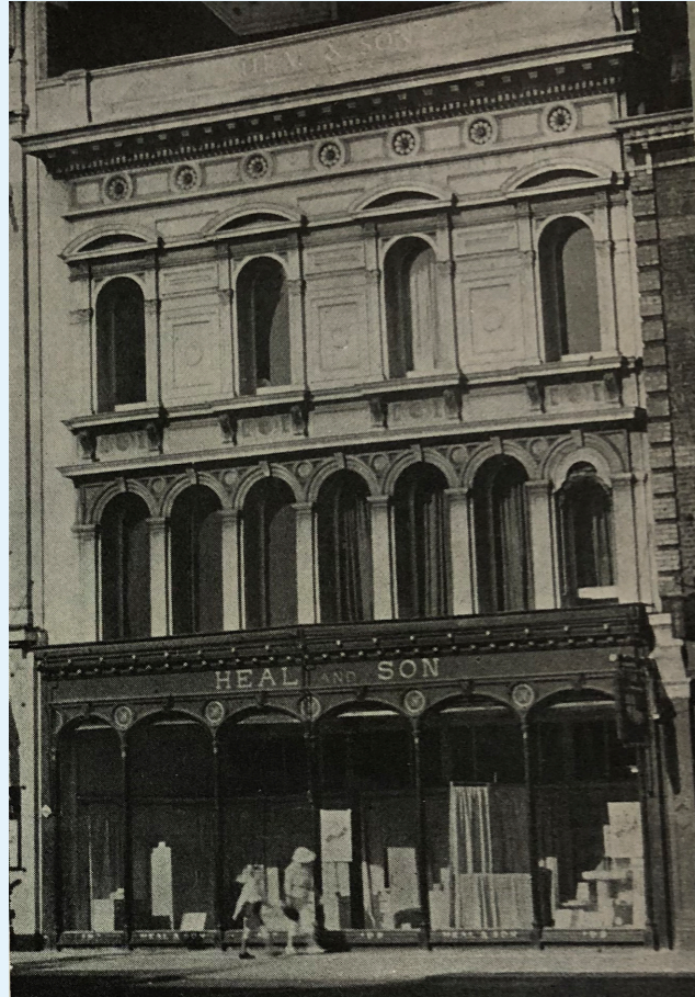
Messrs. Heal's original shop front that was demolished. One of the first buildings to make use of cast iron construction, built between 1854-64.
