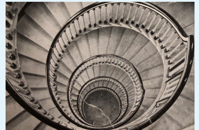
Existing Circular Staircase designed by Messrs. Smith and Brewer for Heal's shop.
