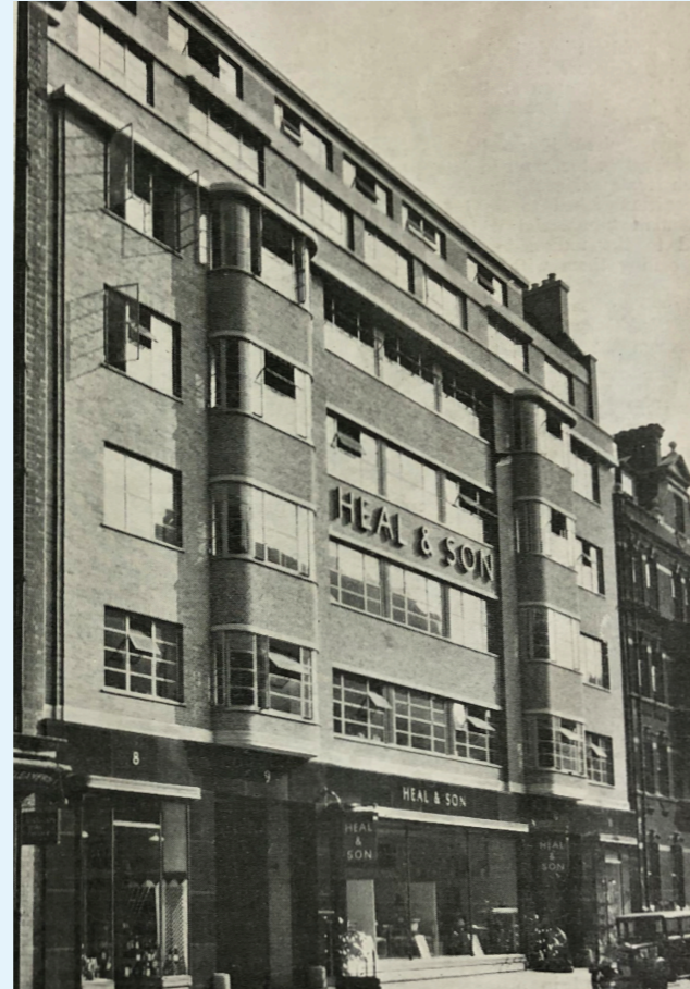
1930s extension to Messrs. Heal & Son's Ltd originally designed as a principal goods depot, warehouse and workshop accommodation. Steel-framed construction with reinforced concrete floors and roofs.
