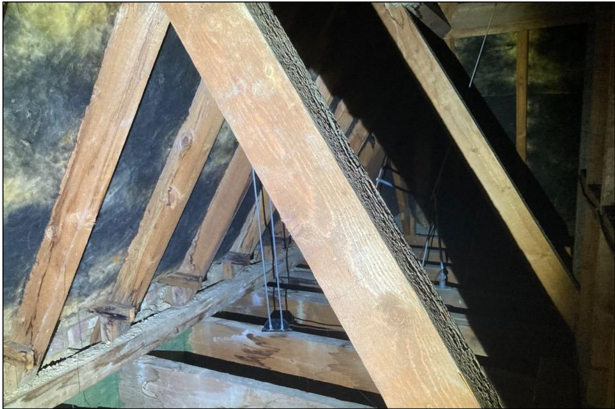
Photograph 4. The small accessible eaves space within the roof of the dwelling.
