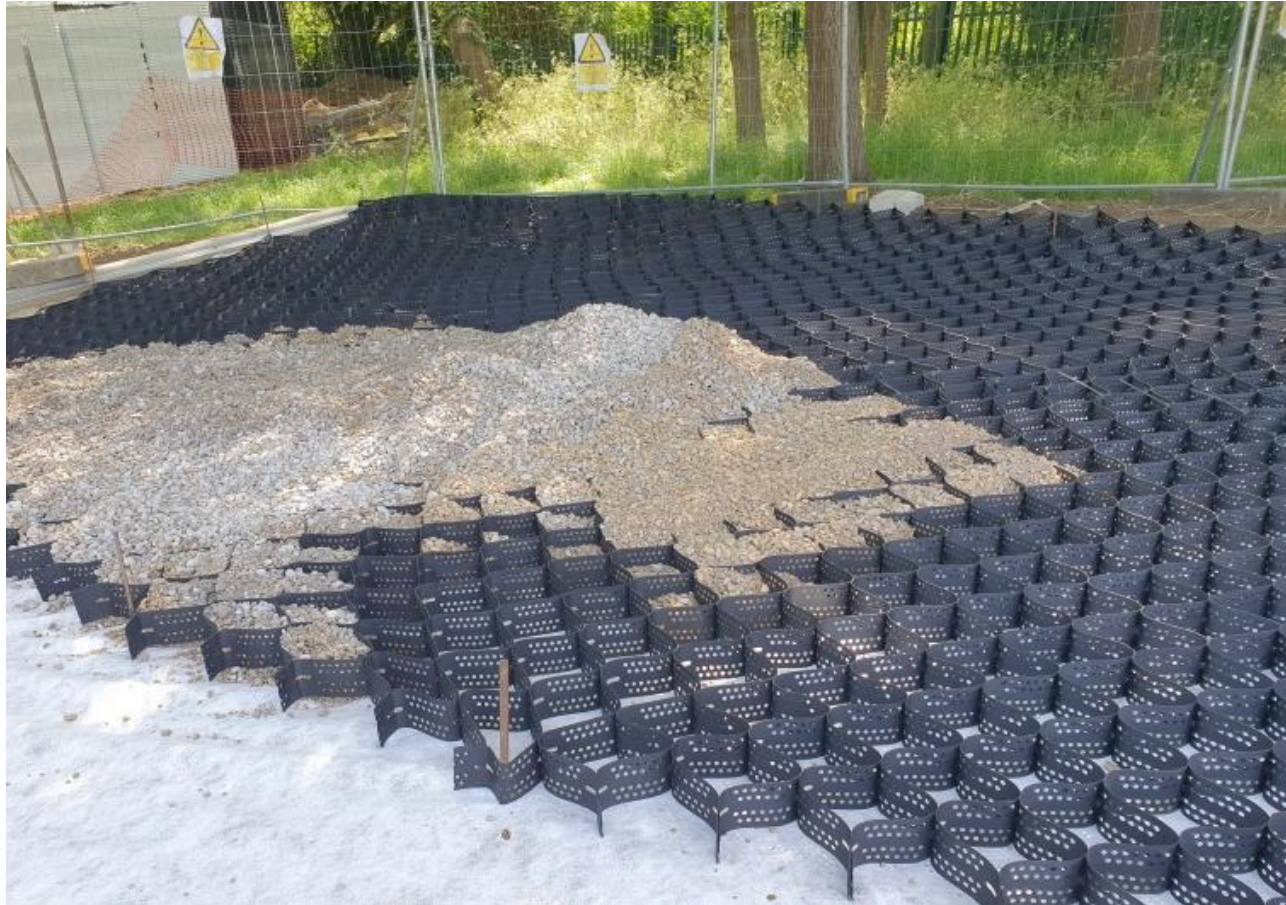
Fig 1: EXAMPLE OF INSTALLATION OF CELLULAR CONFINEMENT SYSTEM
