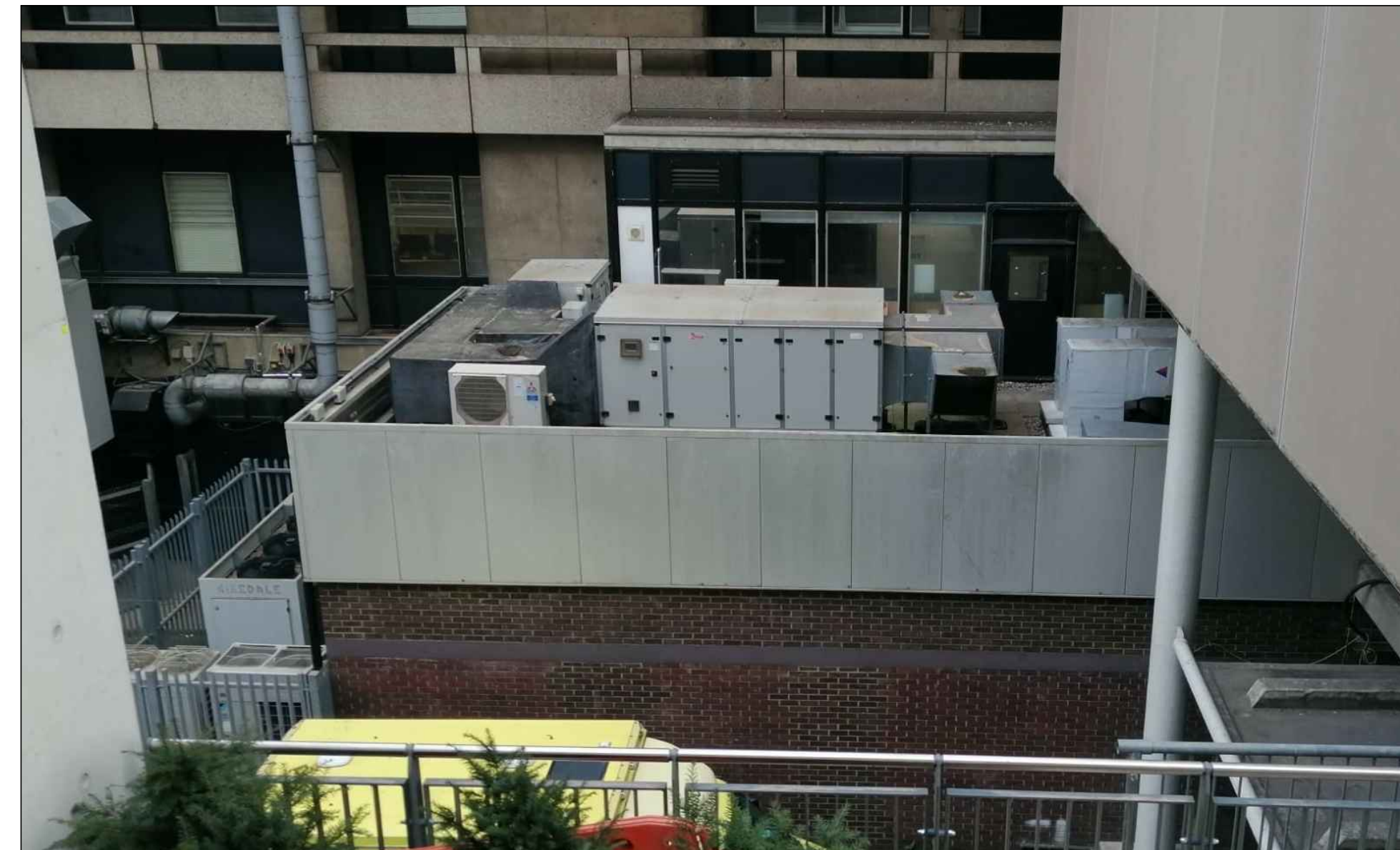
06 Existing Site Photographs (00)003 NTS
