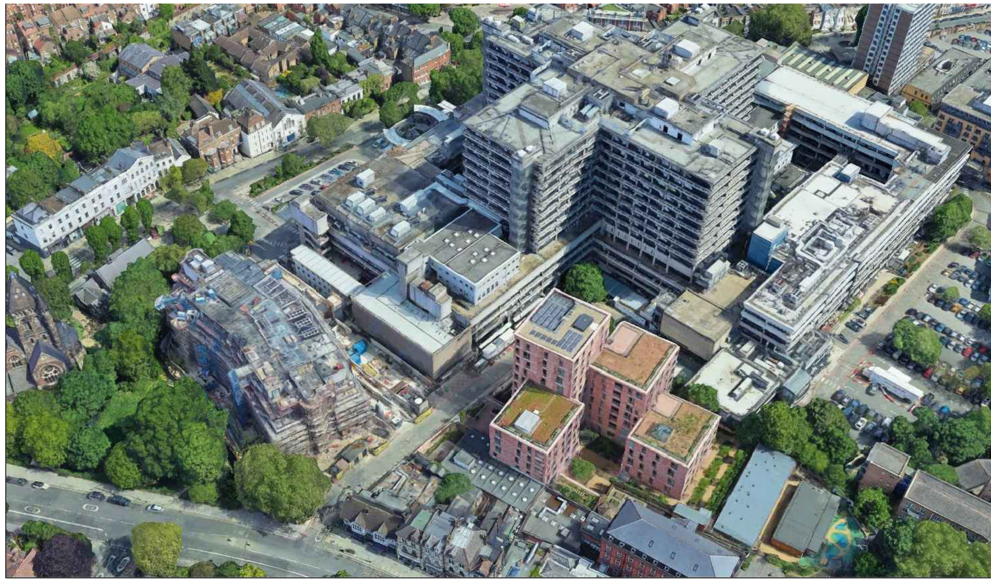
01 Existing Site Photographs (00)003 NTS
