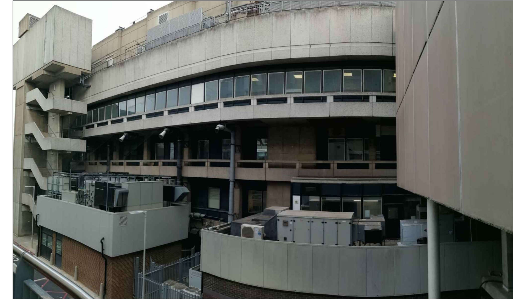
04 Existing Site Photographs (00)003 NTS
