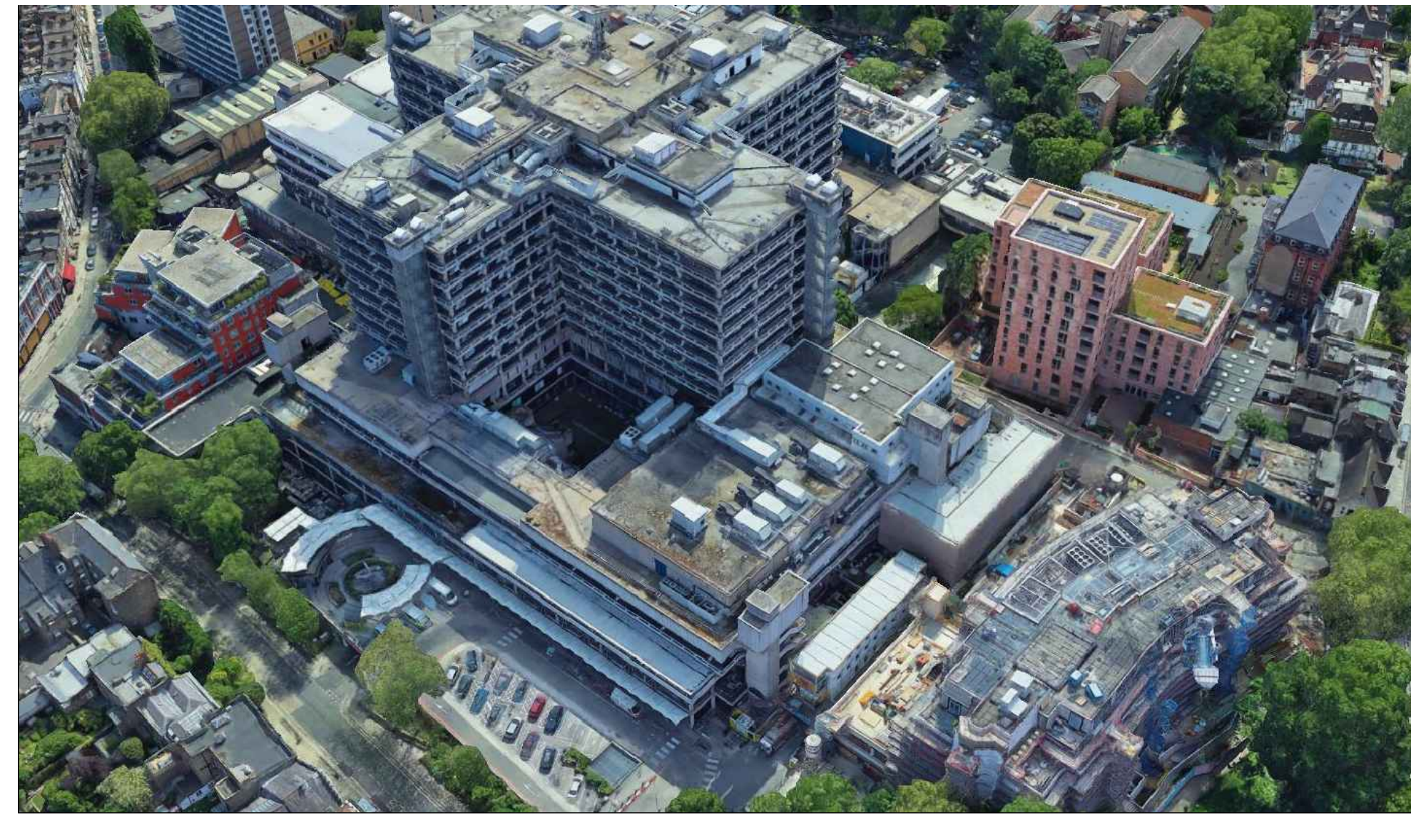
02 Existing Site Photographs (00)003 NTS
