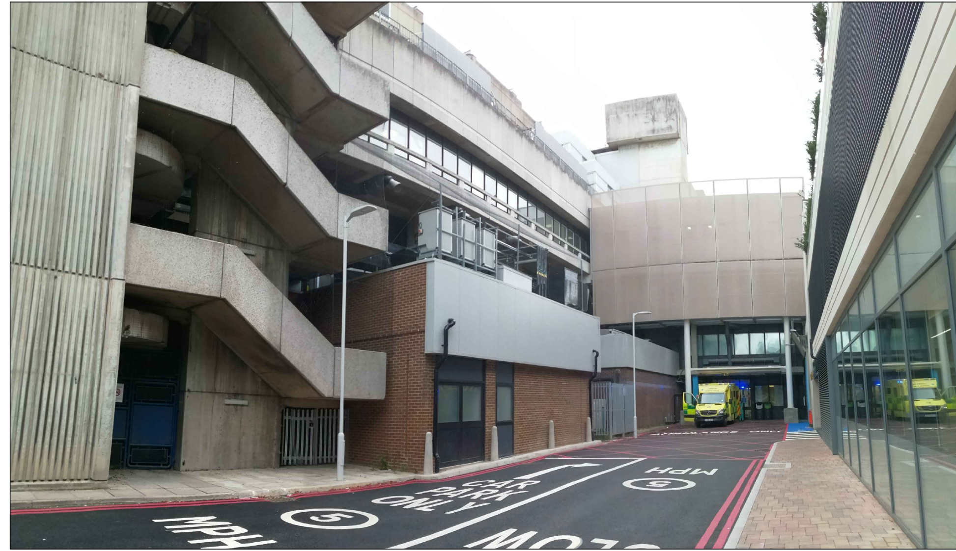
03 Existing Site Photographs (00)003 NTS
