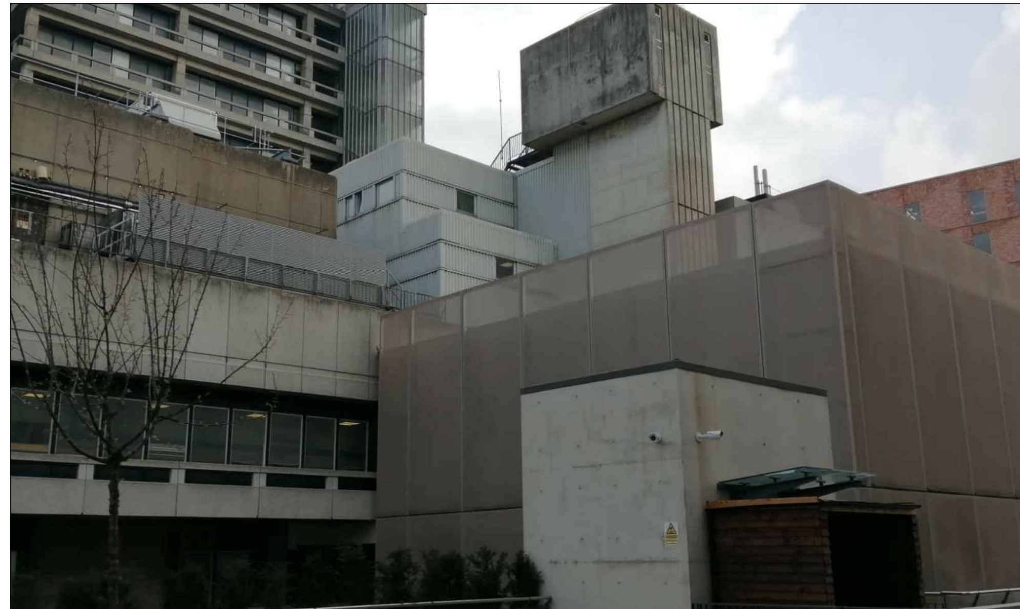
05 Existing Site Photographs (00)003 NTS
