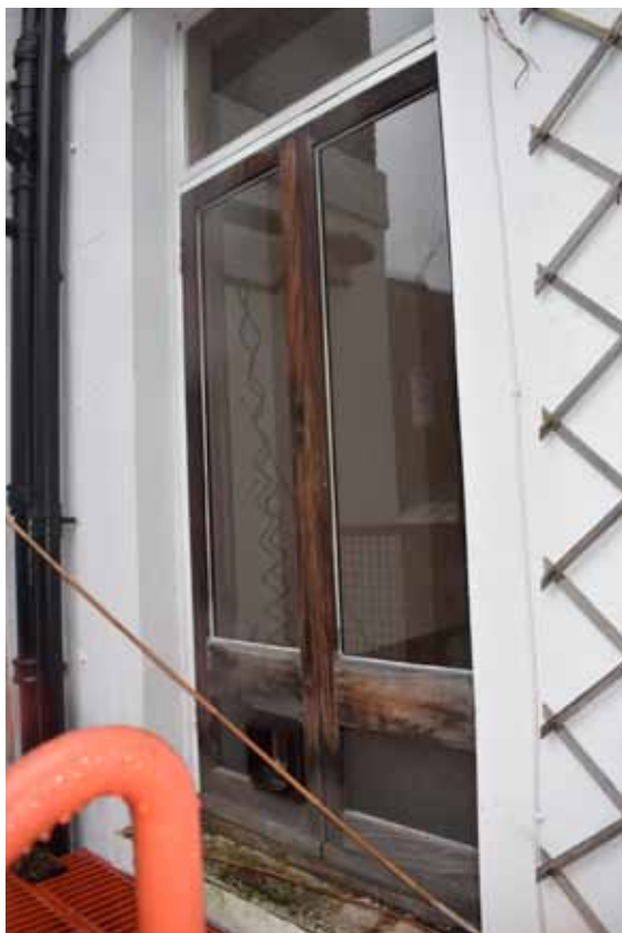
Off balcony : french doors replacing original sash window.
