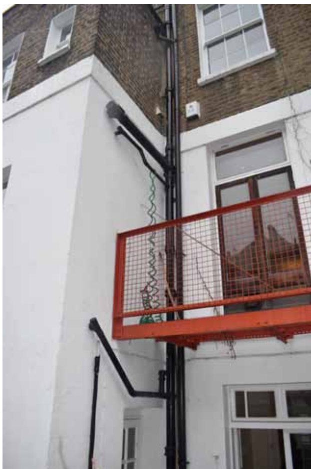
Soil and rainwater pipes along rear facade.
