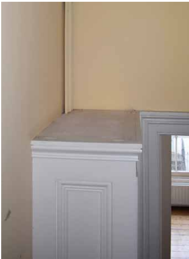
Note modern joinery cut around modern pipework
