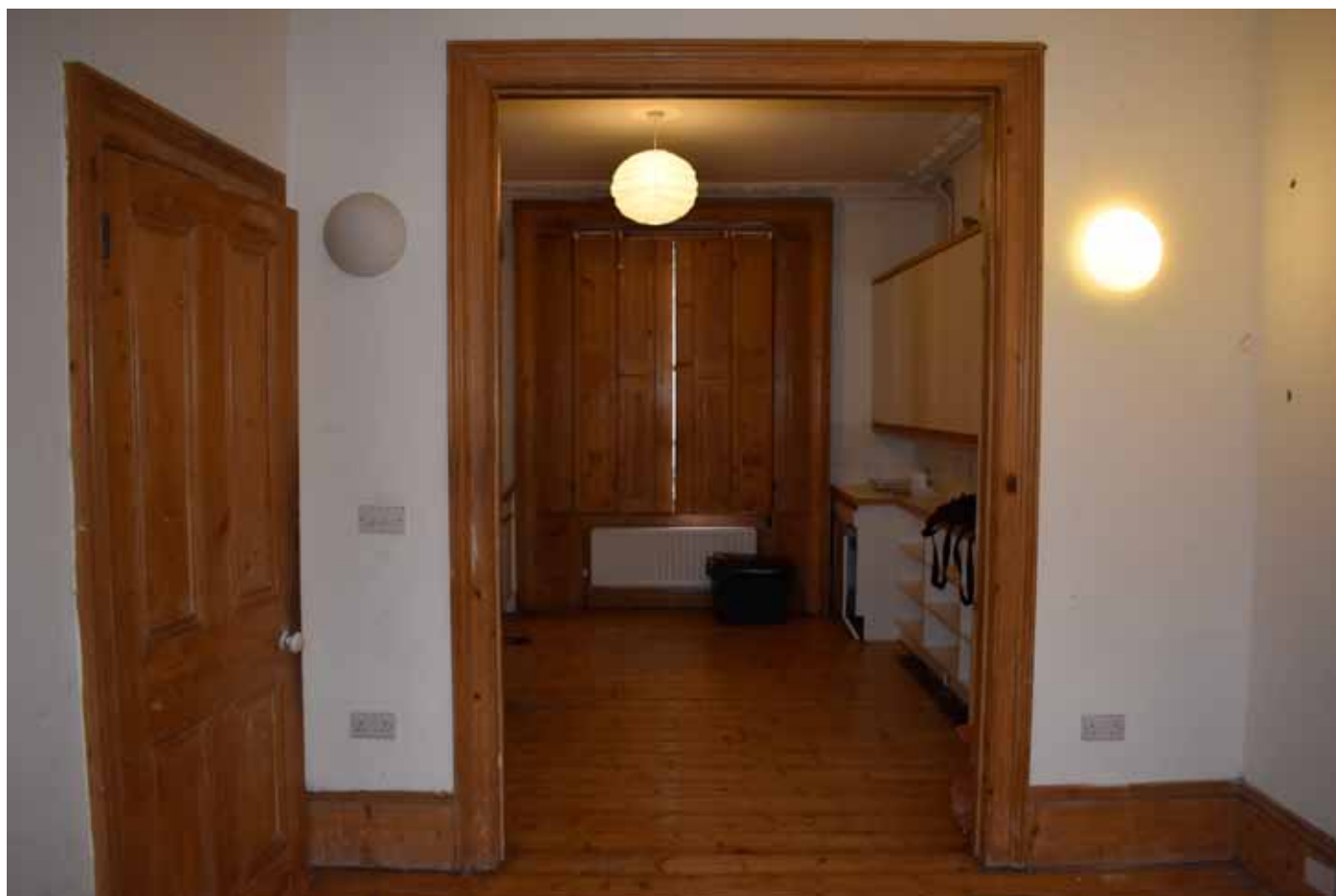
View towards front of house showing original opening: Note double doors missing.
