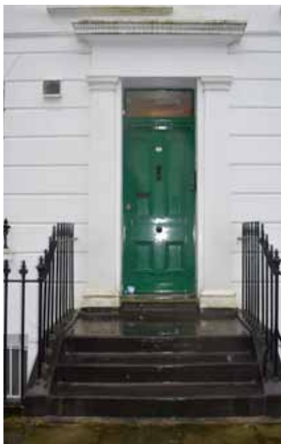
Steps and front Door : Note asphalted steps.
