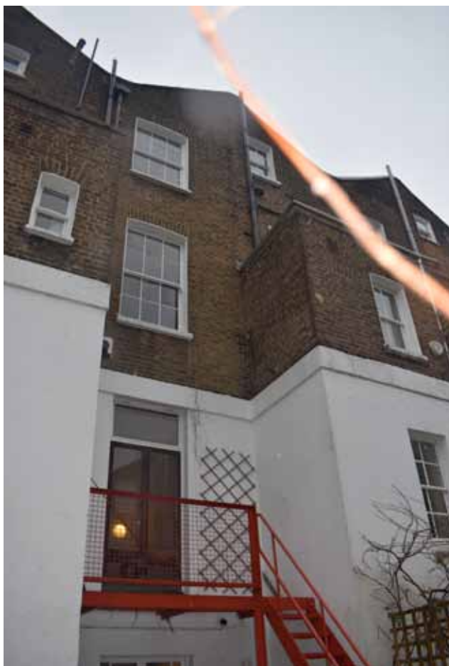
Upper rear facade.:Note projecting asbestos boiler flue at high level.
