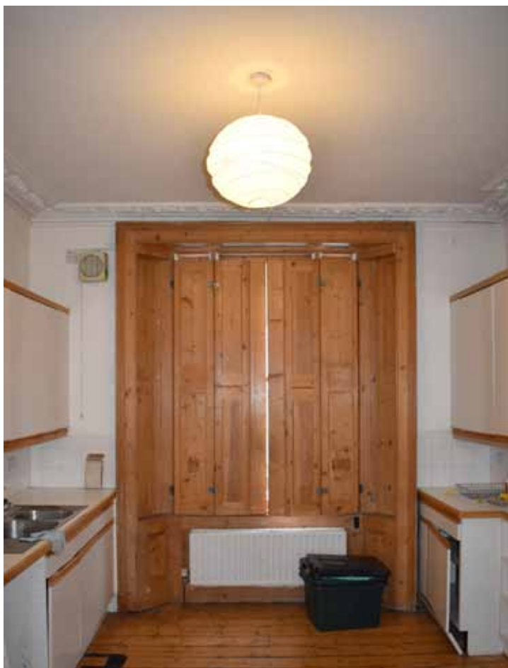
View towards window : Note original shutter box. Ceiling is modern with reproduction cornice, ceiling rose missing.
