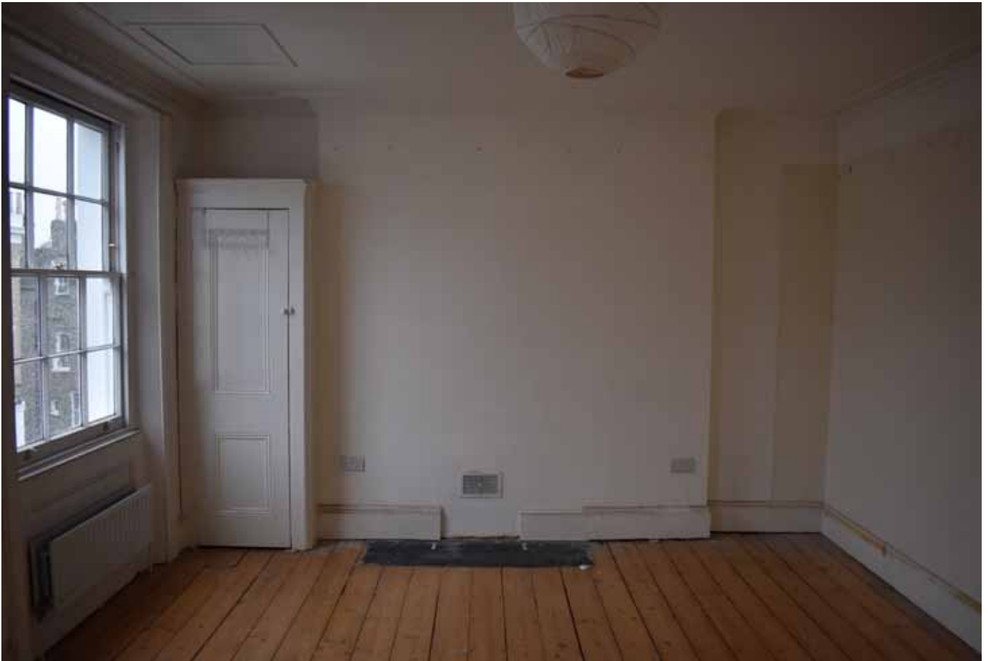
View of chimney breast : Note fireplace missing.
