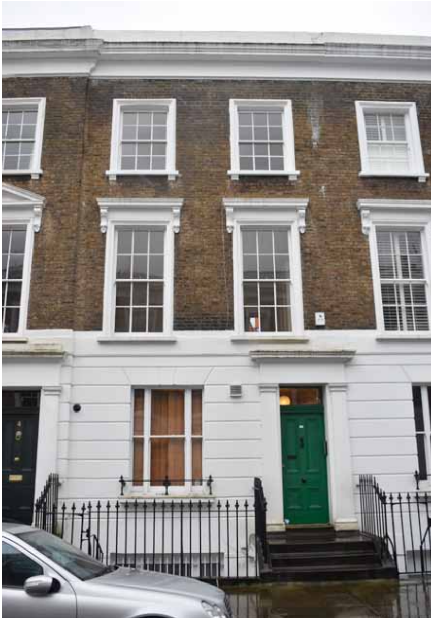
Front View : Note kitchen extract grill, boiler flue and missing brackets to cornice.
