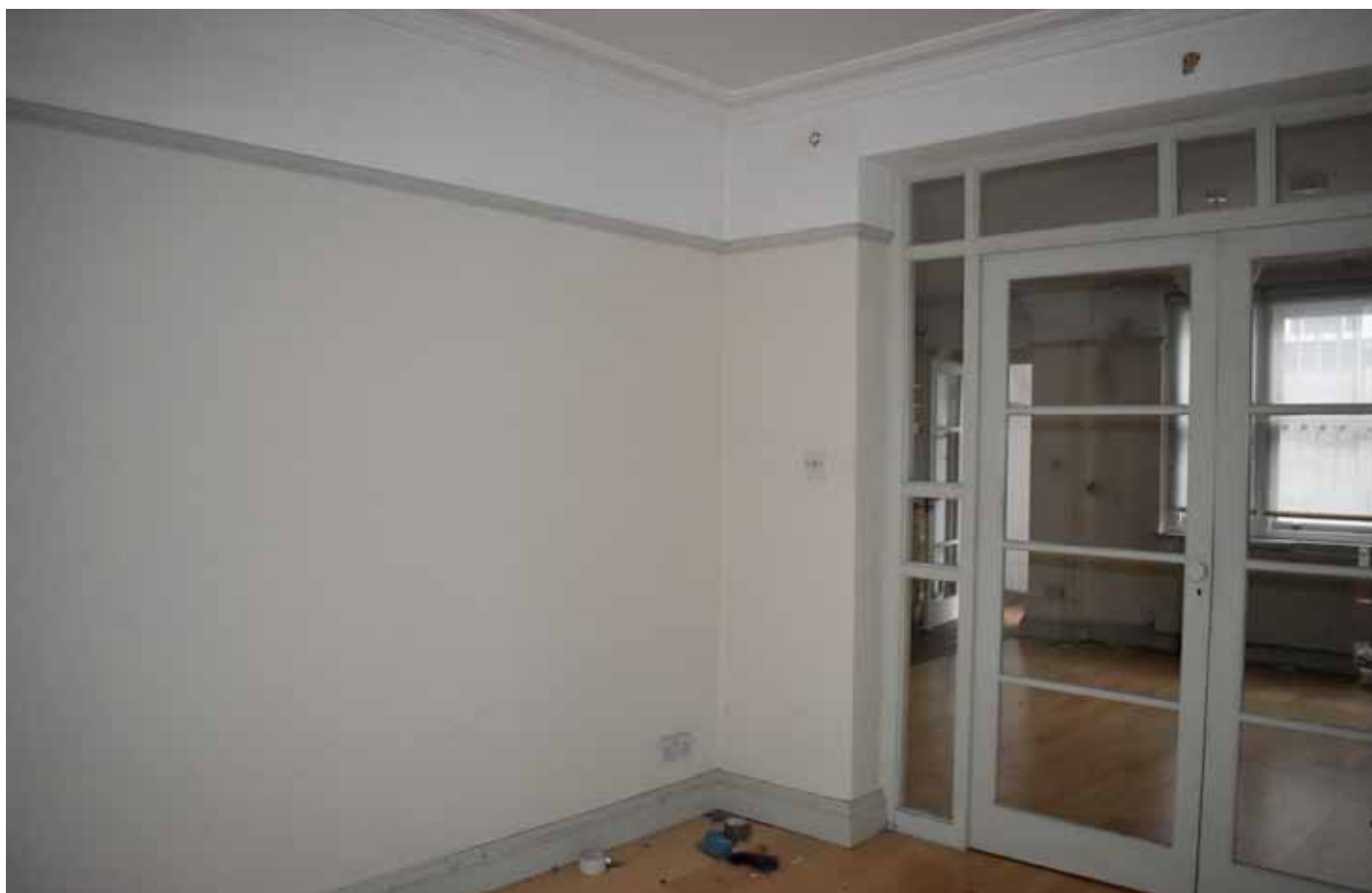
View from rear room towards spine wall showing modern opening
