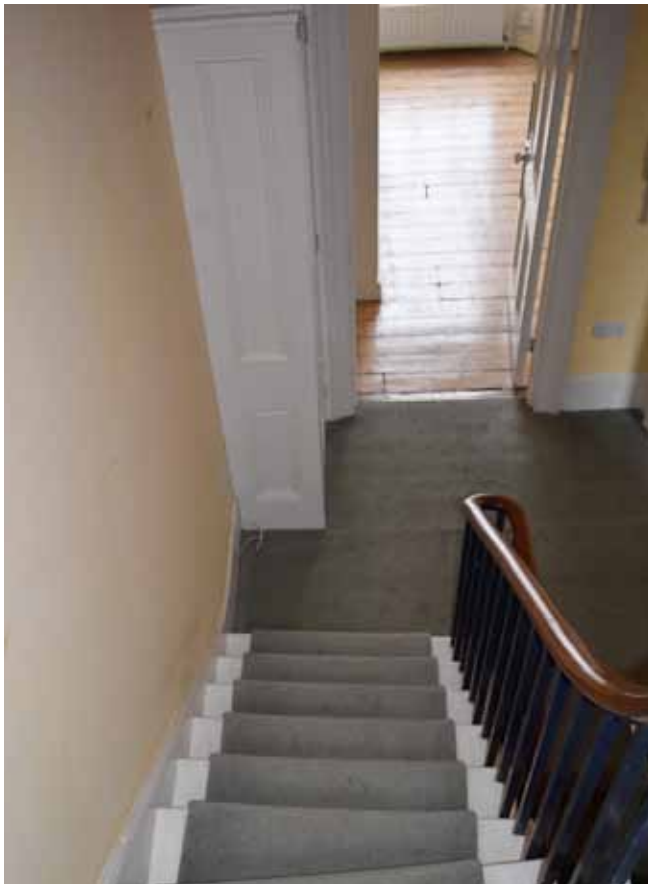
Note modern joinery cut around original skirting
