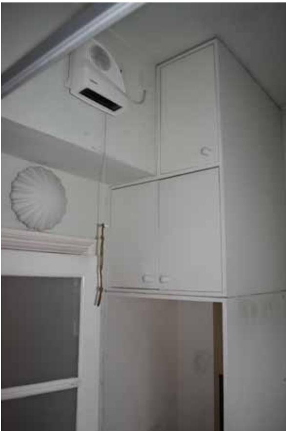
Door to hallway : Note modern boxing out and modern door to original frame.
