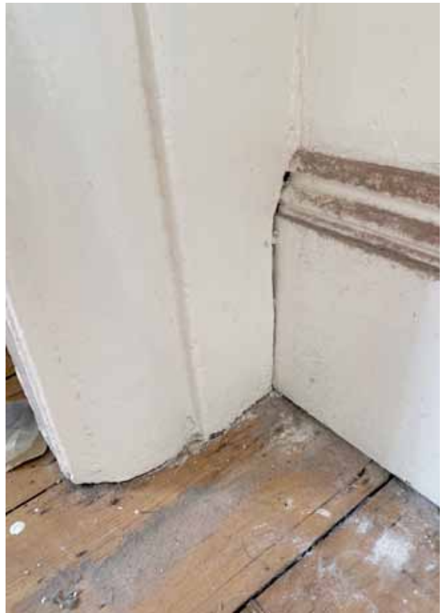
Cupboard joinery cut around skirting
