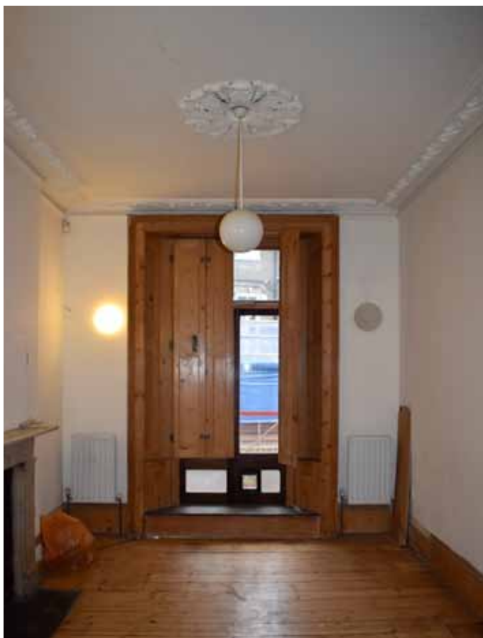
View toward window : Note modern french doors and missing bottom section of shutter box.
