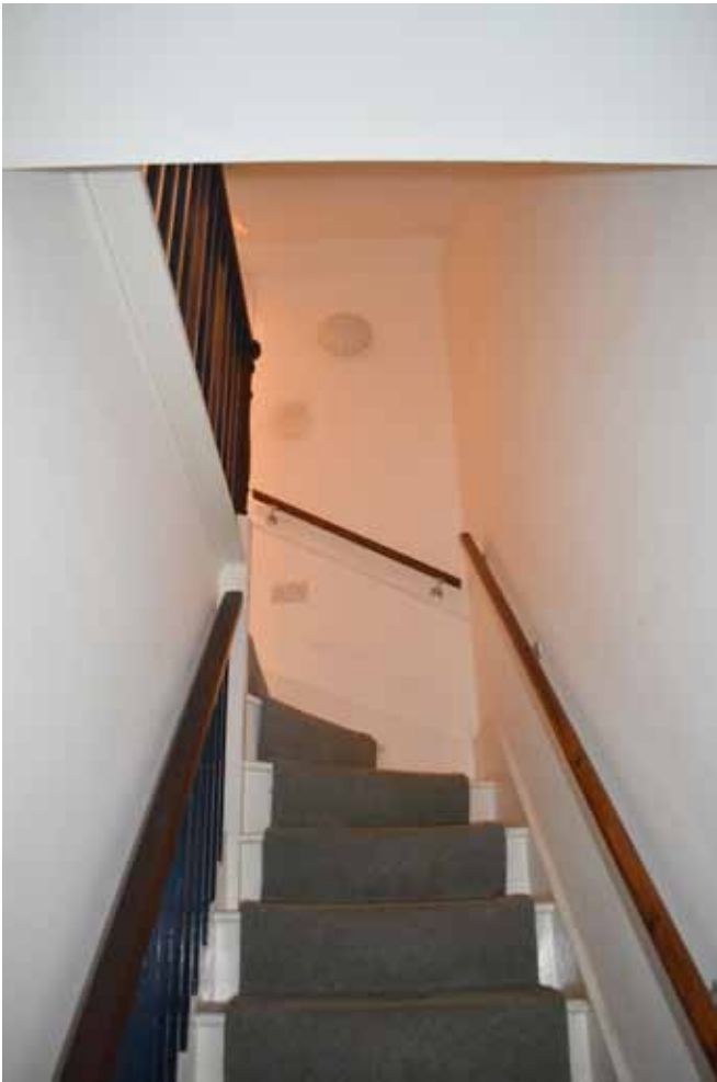
Staircase to basement : Note modern stair and wall dividing old hallway
