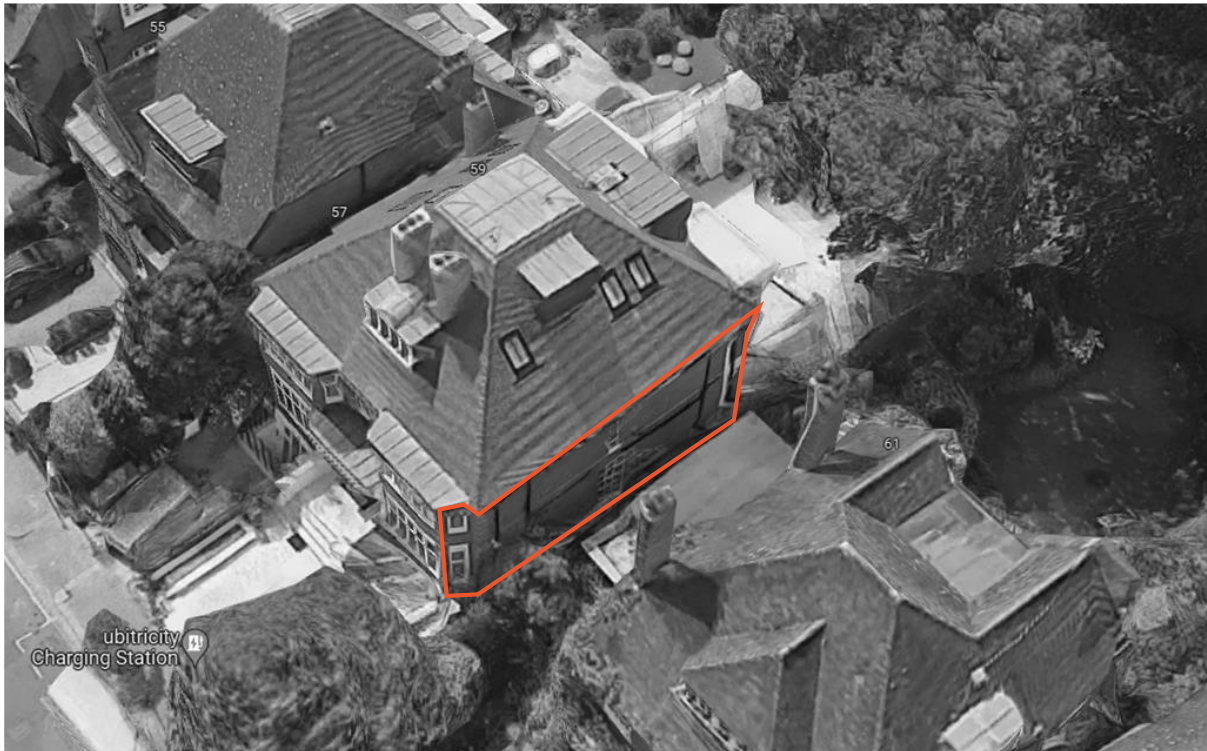
Figure 6: Image of the building assessed at 59 Redington Road
