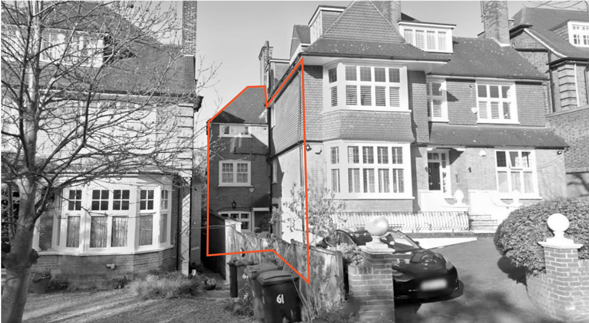
Figure 7: Image of the building assessed at 63 Redington Road
