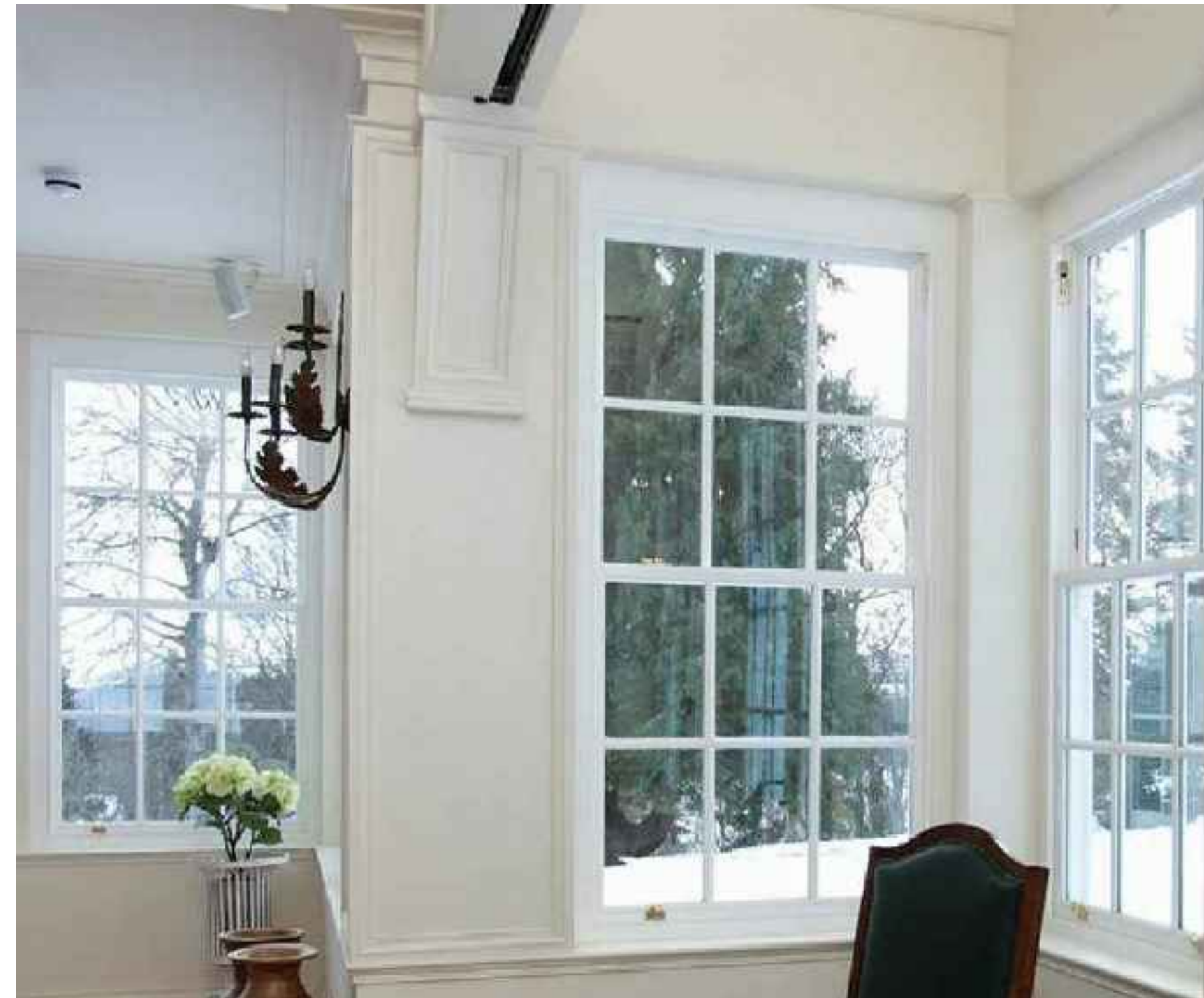
Spec: New painted timber sliding sash window Supplier: Bereco or equal Finish: Matte finish, painted timber Colour: White
