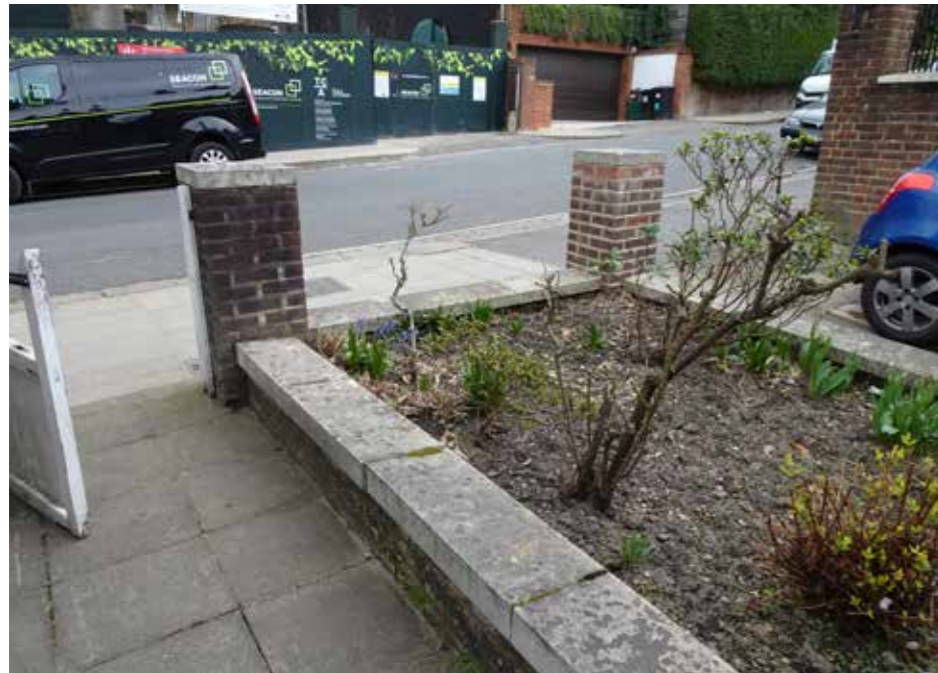
Above: Existing planting and soil condition is very poor. The landscaping is overly dominated by the large 1960's coping stones which are visually heavy.
