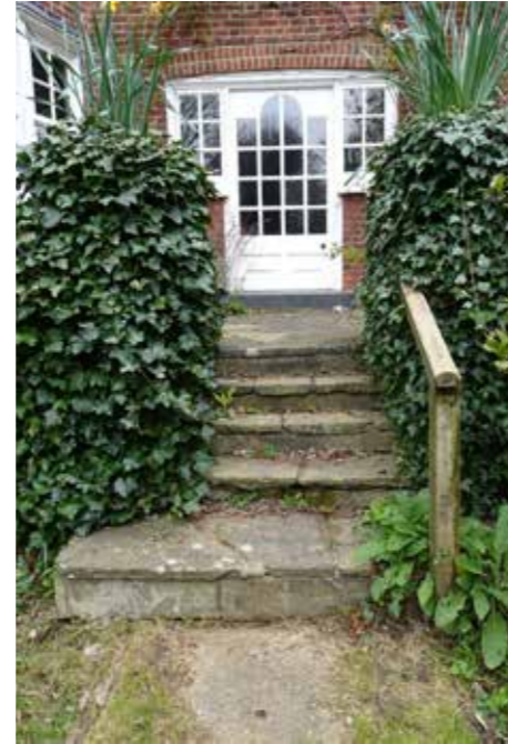
Above: Existing steps from the 1960's formed in broken concrete paving.
