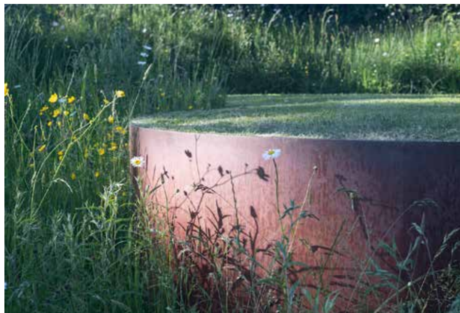
Bespoke cor-ten steel edging is used to maximise the overall planting area by avoiding heavy brick upstands.
