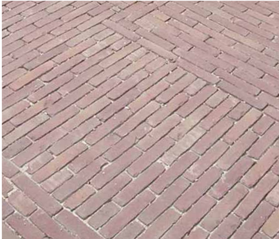
Vande Moortel Mahogany red tumbled unsanded clay pavers laid in a stretcher pattern to the long walk and new paths, fully permeable.
