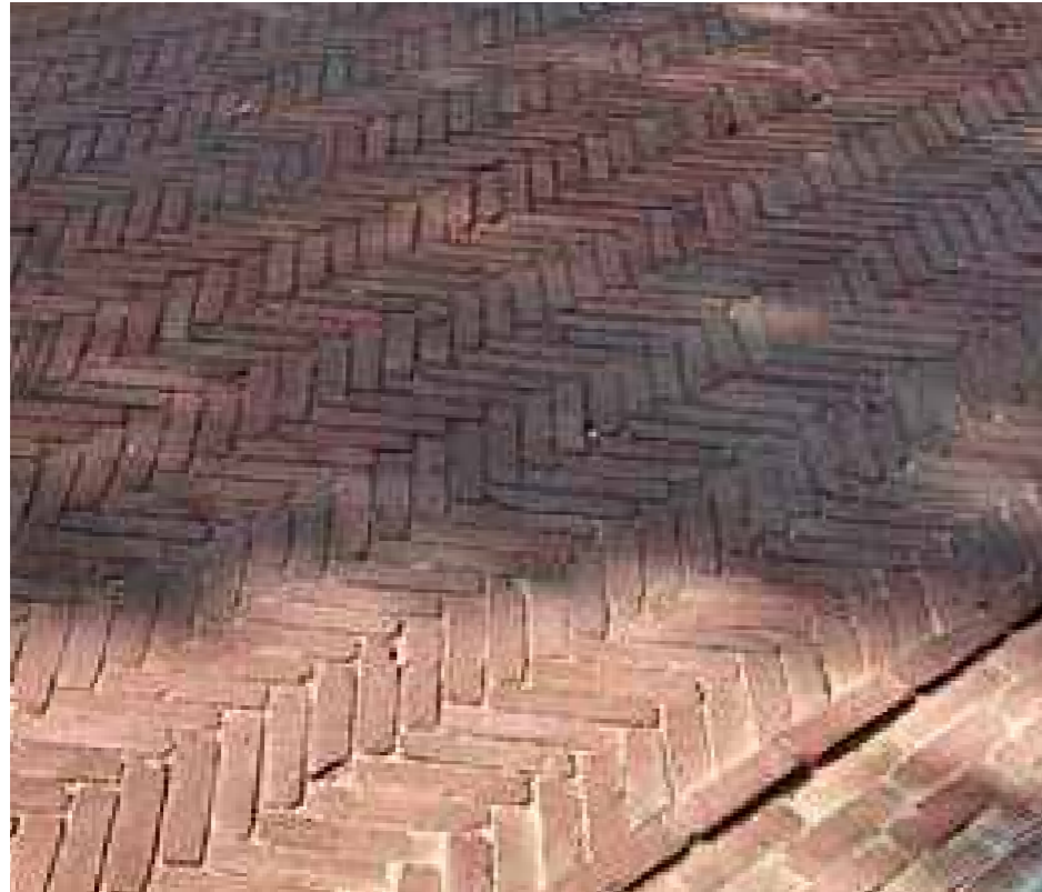
Vande Moortel Mahogany red tumbled unsanded clay pavers laid in a herringbone pattern.
