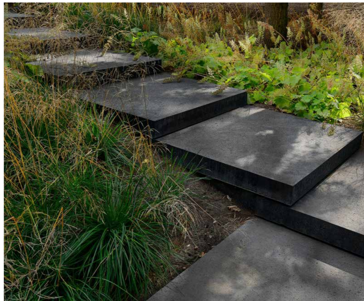
Large scale Black-Basalt stone effect pre-cast units by Schellevis form the cascade of steps and planting to the new entrance.
