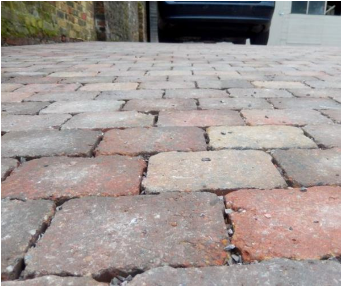
Photo: An example of a finished permeable block paved driveway
