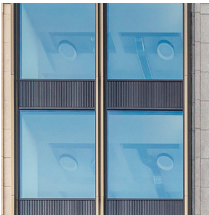
Spandrel panel detail / Frame surround
