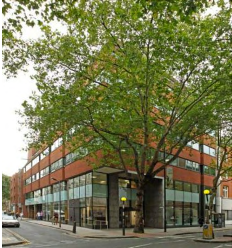
Figure 1: 164 Shaftesbury Avenue; Mercer Street is on the left
