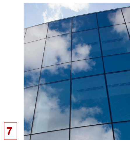
7 Curtain wall with silicone joint
