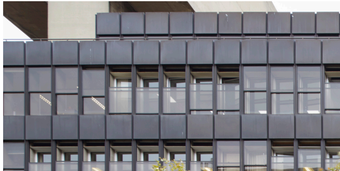
Existing aluminium glazed facade
