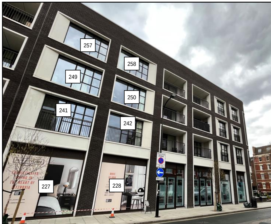
115 to 125 Cleveland Street
