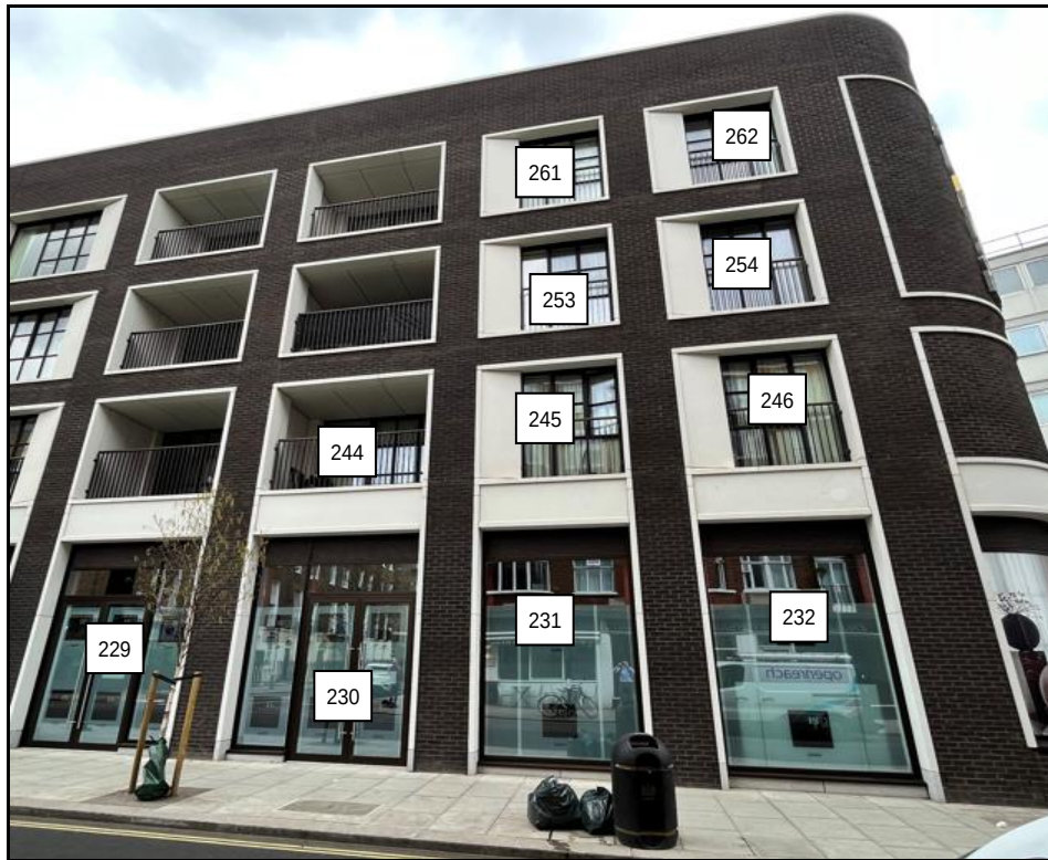
115 to 125 Cleveland Street
