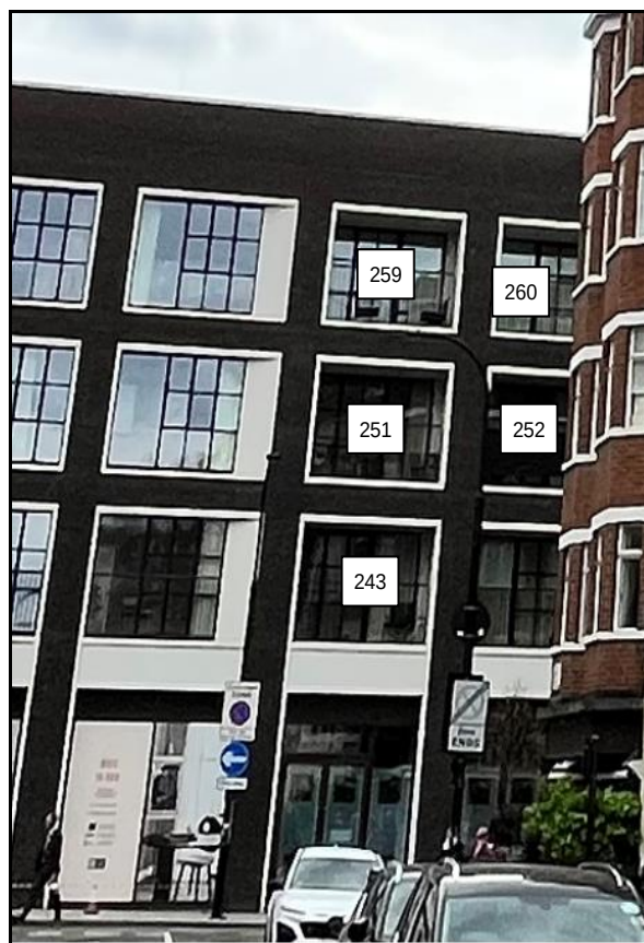
115 to 125 Cleveland Street
