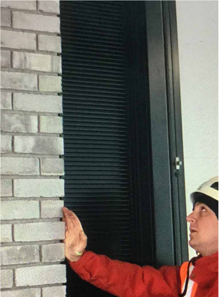
Intake louvre as installed
