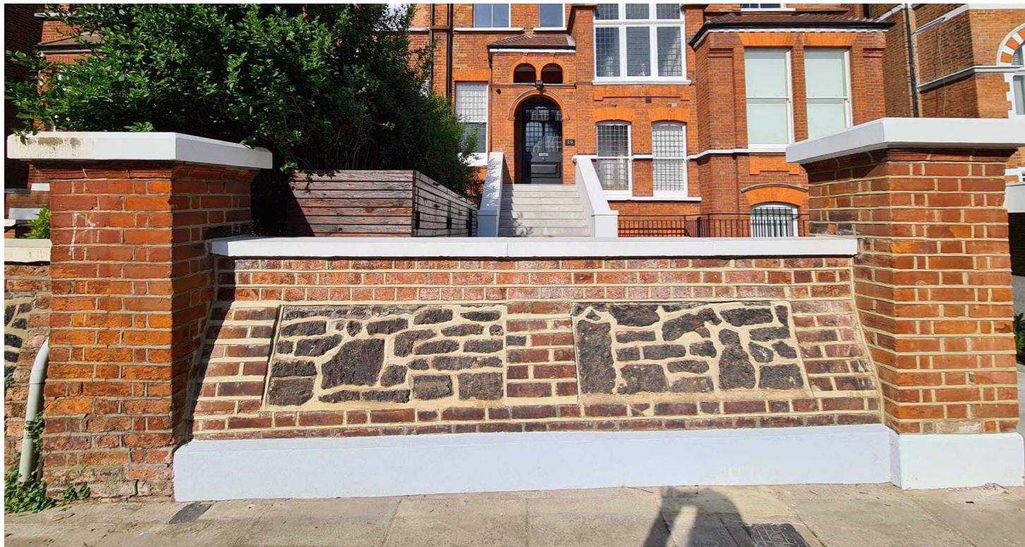
Fig 10. The front brick wall and piers were cleaned and repointed
