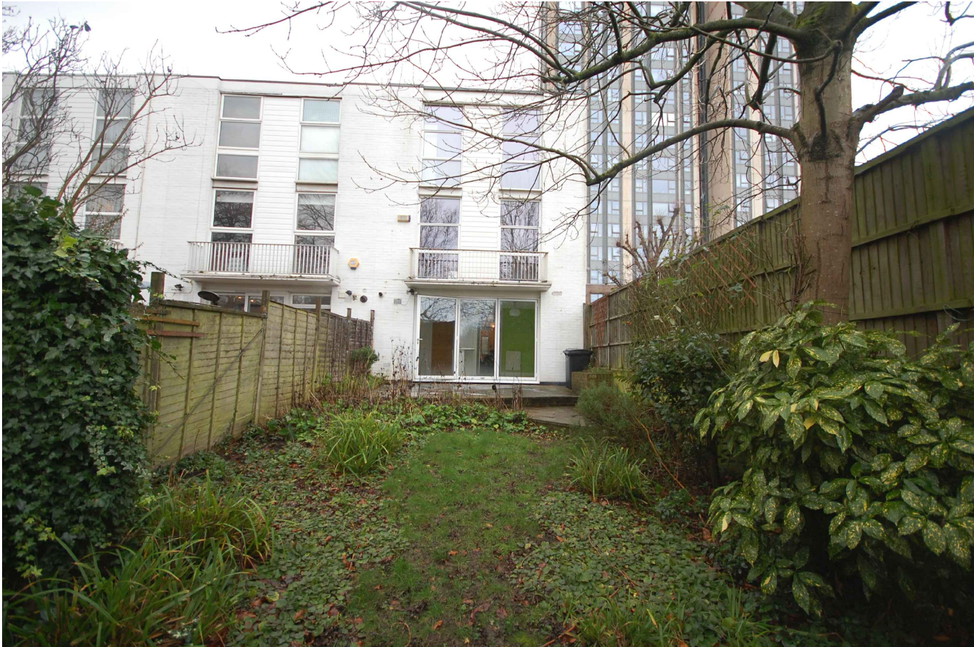
REAR ELEVATION FACING SOUTH
