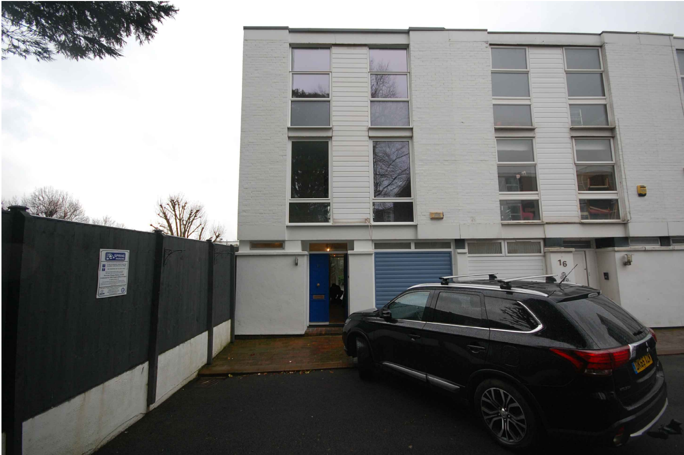
FRONT ELEVATION FACING NORTH
