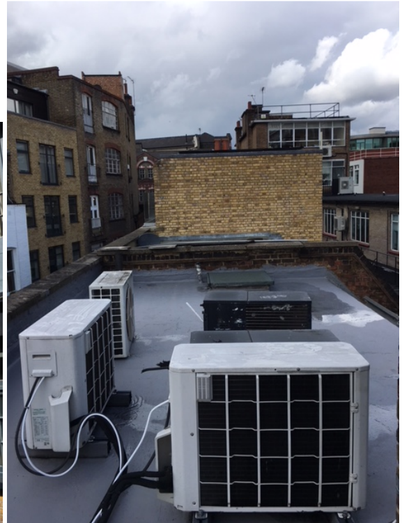
2. Rooftop looking north to extension on no. 9
