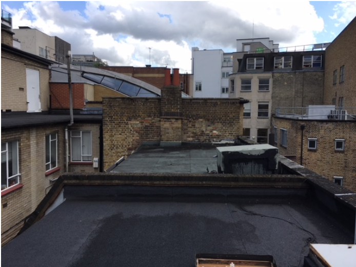
3. Rooftop looking south
