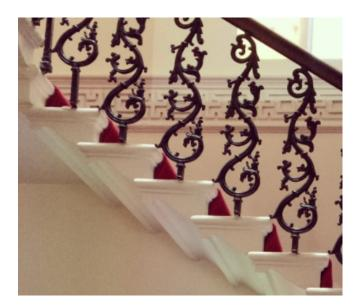
A second stair (Stair 1) connects Ground and Basement levels and offers reasonable access. Stair lighting will be upgraded with integral LED strips in handrails.
