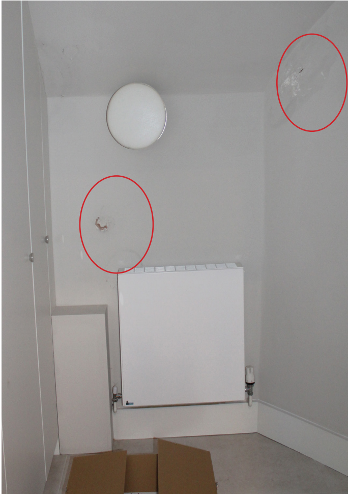
Figure 3: Internal damp
