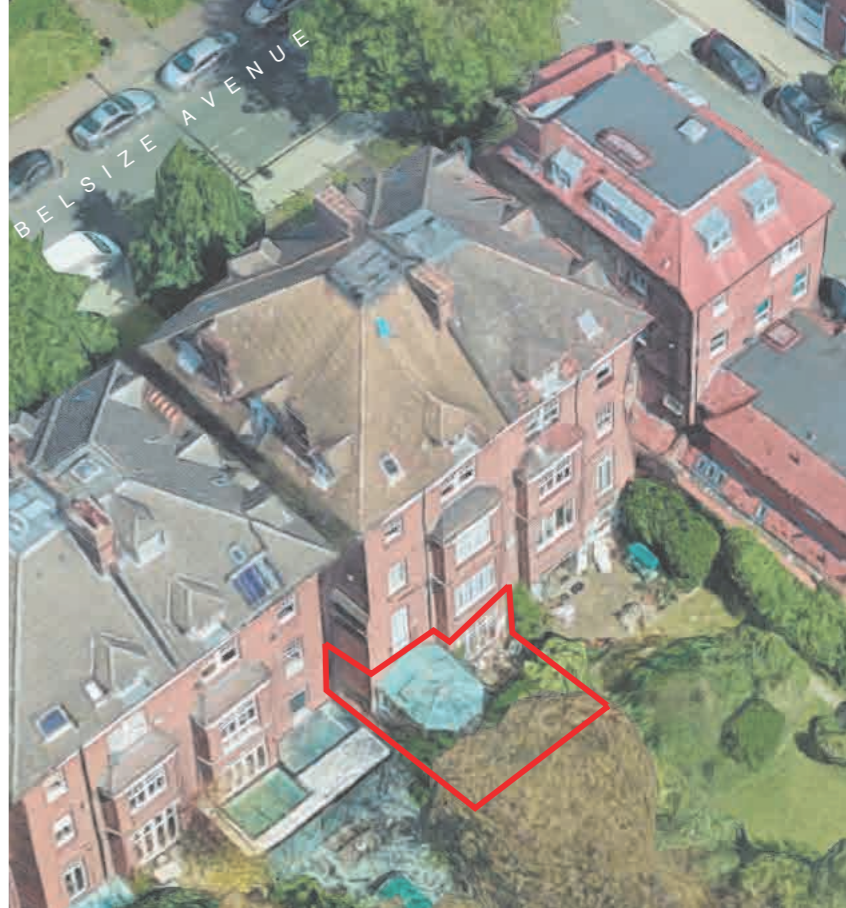
Site aerial view, looking east
