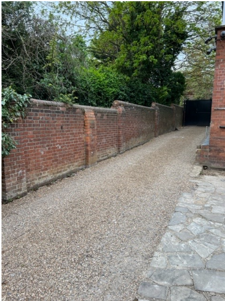
View of the boundary wall across the access driveway
