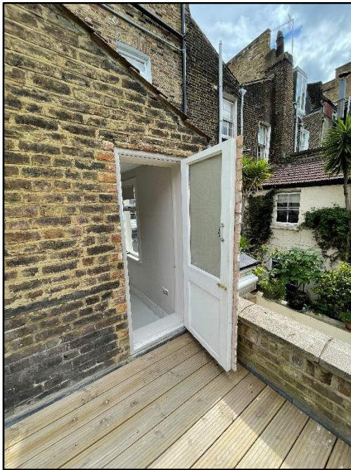
Figure 1 – Photo of single width door providing access to the flat roof.
