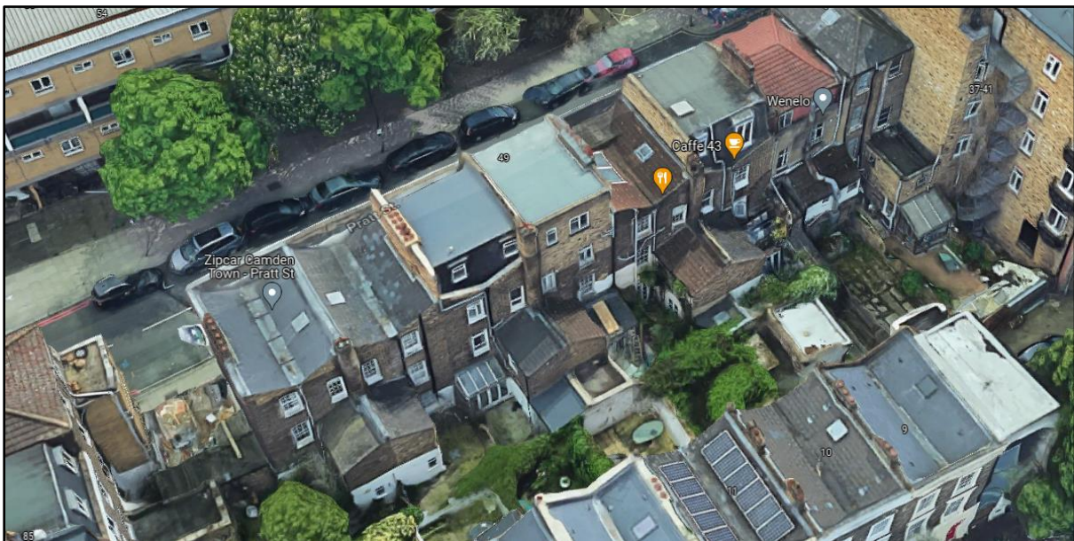
Figure 3 – Rear elevation of terrace within which No. 49 sits. Note variety in rear extensions, roof forms, outbuildings and rear curtilage surfacing and boundaries.
