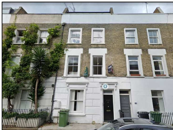
Figure 1 – Front façade of 49 Pratt Street
