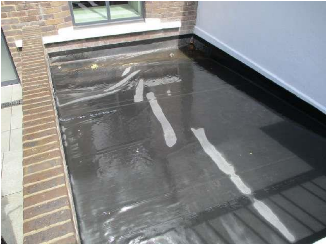
3. Photo showing Roof B.
