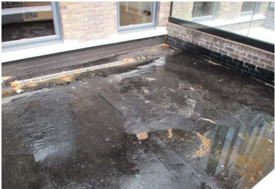
4. Photo showing Roof A.
