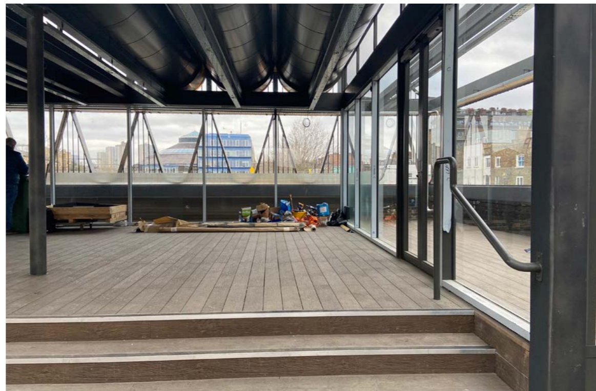
Existing entrance view on terrace
