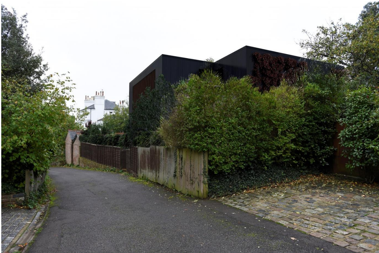
AS PROPOSED – CANTILEVERED FIRST FLOOR SET BACK FROM MILLFIELD PLACE BY 1.75M TO RESPECT THE BUILDING LINE SET BY THE HOUSE AT 1 MILLFIELD PLACE. VERTICAL LOUVERS TO AVOID VIEWS
