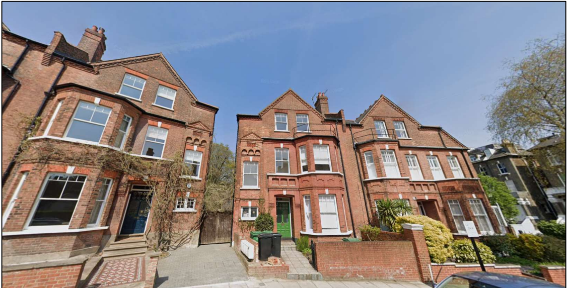
Figure 2.2: Front Elevation of the Site (from Downside Crescent)
