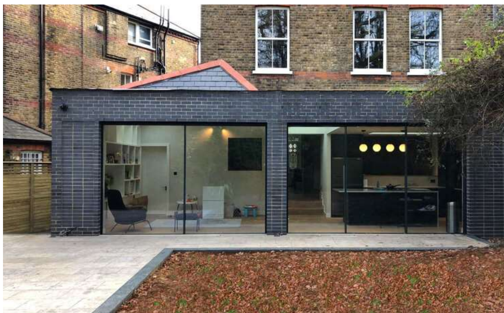
[Photo above: The full width extension of the adjacent property at 31 Downside Crescent. Although the slate roof was reconstructed over the original side of the extension which maintains the architectural history of the building (i.e., the dominance of the original side of the extension), the materials used clearly distinguish the new extension from the original building. At 33 Downside Crescent, the Applicant wishes to use London stock bricks with red-brick decorative coursing which will mean that the extension will harmonise more with the original building.]
