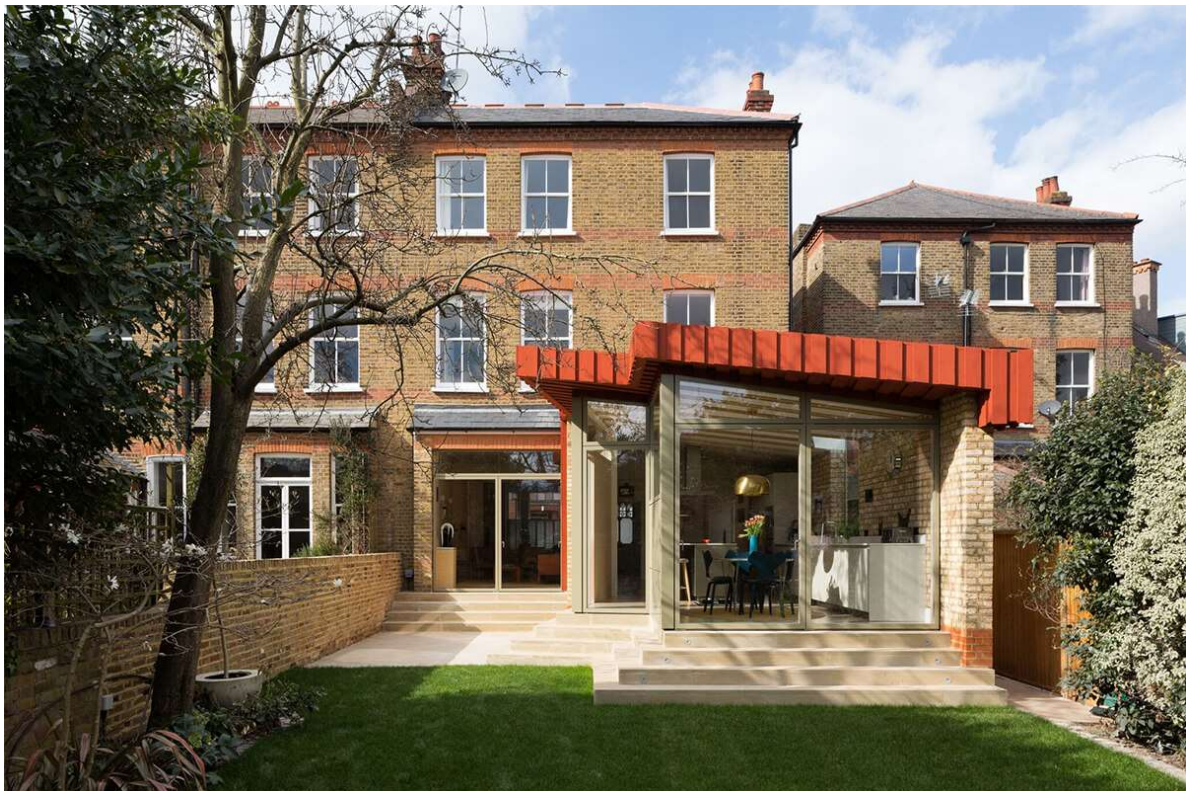
[Photo above: The extension at 4 Downside Crescent.]
