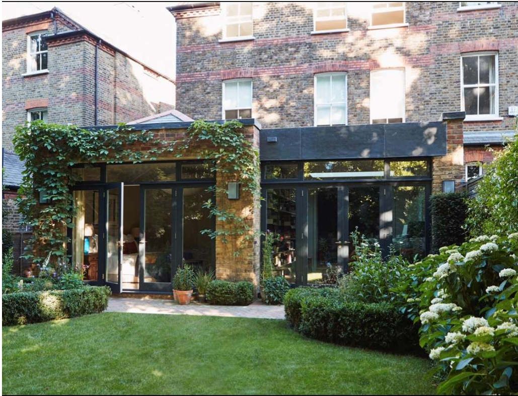
[Photo above: The full width extension at 27 Downside Crescent. This is an example of a successful full width extension on this street using traditional materials which relate to the original property. The dominance of the original extension was maintained by re-constructing a slate pitched roof with red terracotta tiles on the corners over the original side, with a flat roof over the “infill”. Traditionally designed timber framed windows and doors complete the authentic period appearance of this extension: design elements which we have been inspired to replicate at the scheme at 33 Downside Crescent.]
