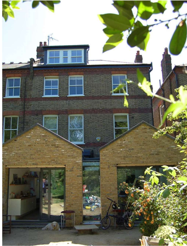
[Photo above: The full-width extension at 5 Downside Crescent which uses more traditional brickwork than the darker bricks used at 31 Downside, but this example has two “peaked” roof lines over the original side extension and the new “infill” which means it has lost the architectural history of retaining a dominant side in the location of the existing extension.]
