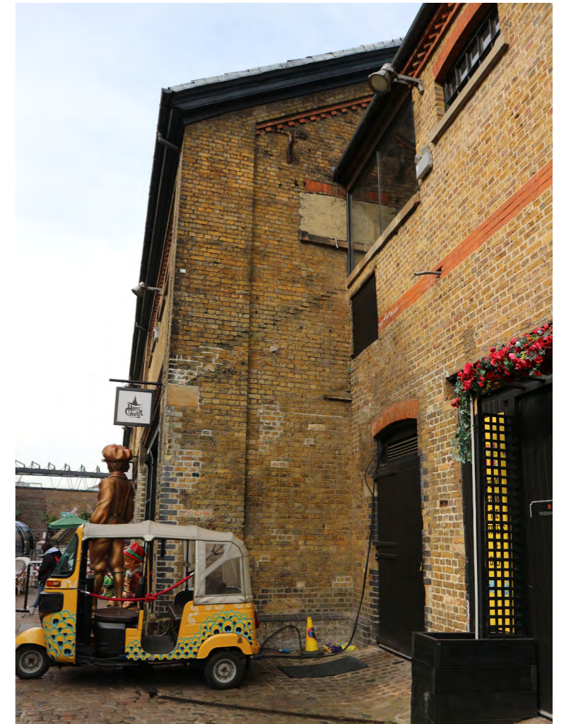
3.3 East Elevation of 1882 stable
