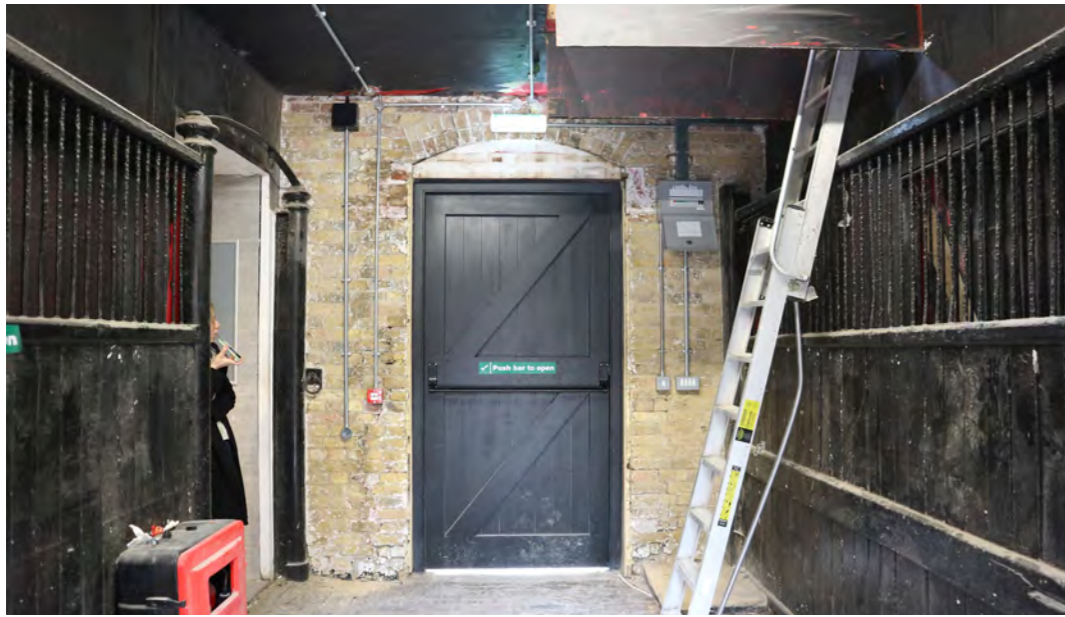
3.10 Entrance Lobby F2
