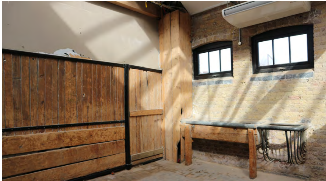
3.11 Loose box at north western corner of stable F4
