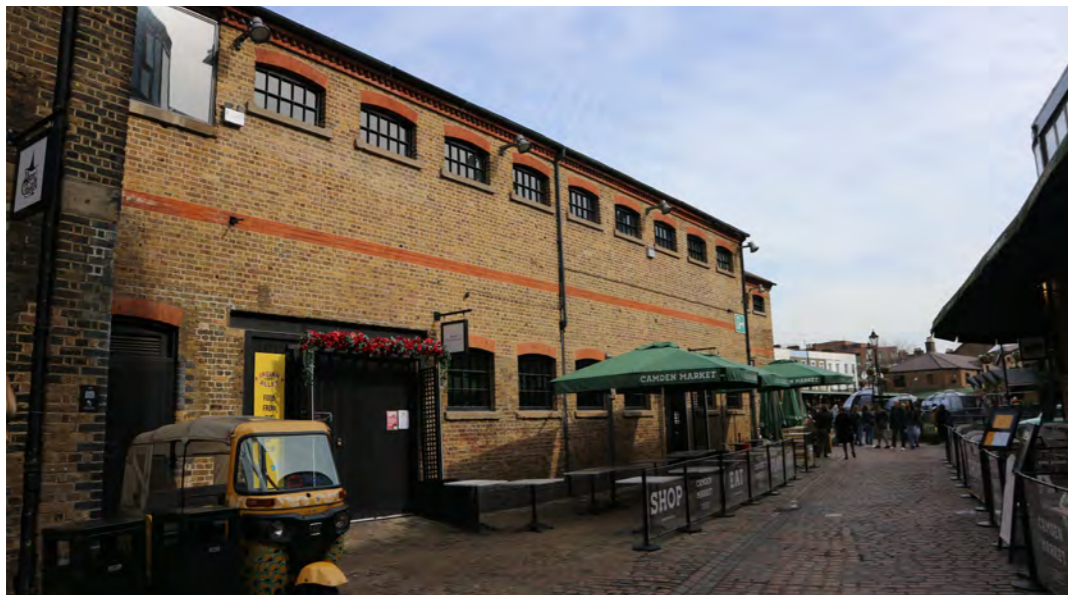
3.4 South Elevation of 1897 stable range
