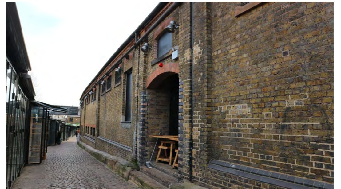
3.8 North elevation looking west, towards the 1897 extension
