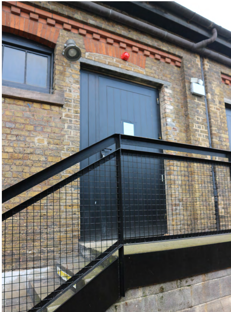
3.7 Doors and Concrete extension on North elevation
