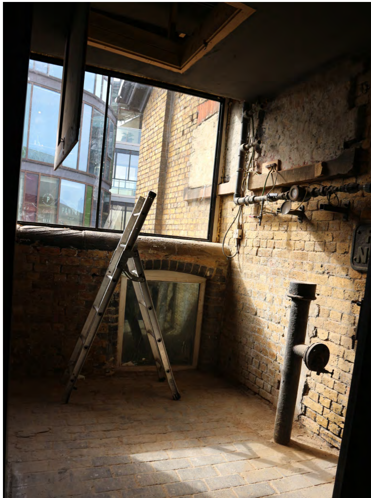
3.20 Modern window insertion F16
