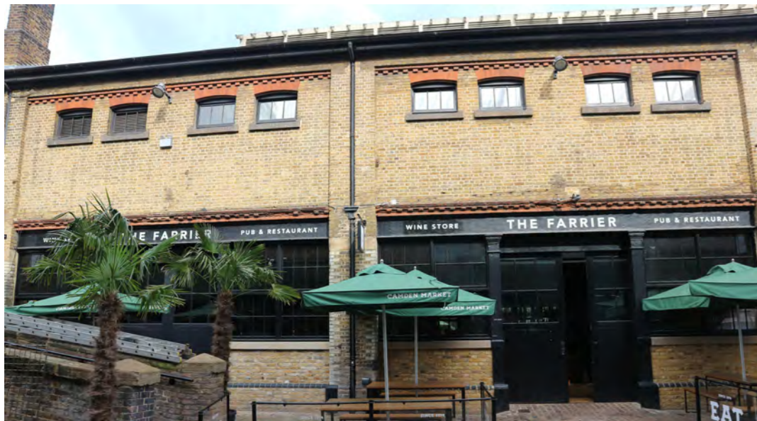
3.2 South elevation of 1883 building
