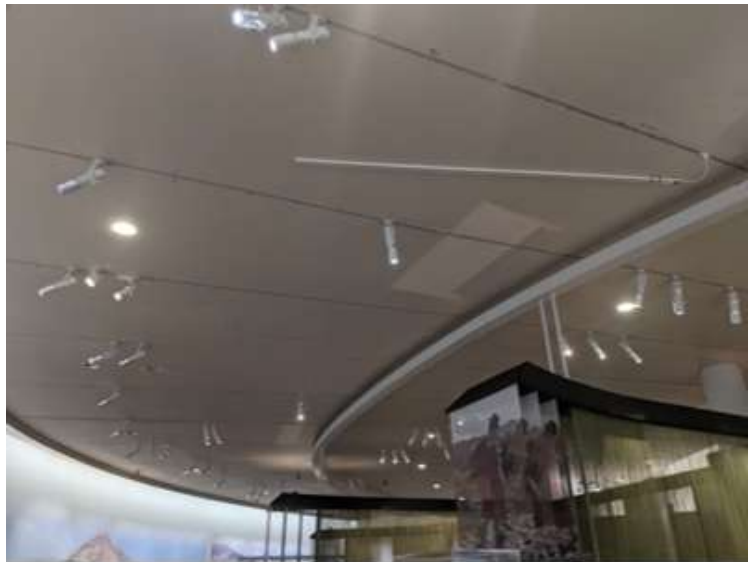
Above: existing ceiling, recessed lighting track and surface mounted fixtures to painted plasterboard ceiling. Left: existing cork floor tile finish, with inset floor box
