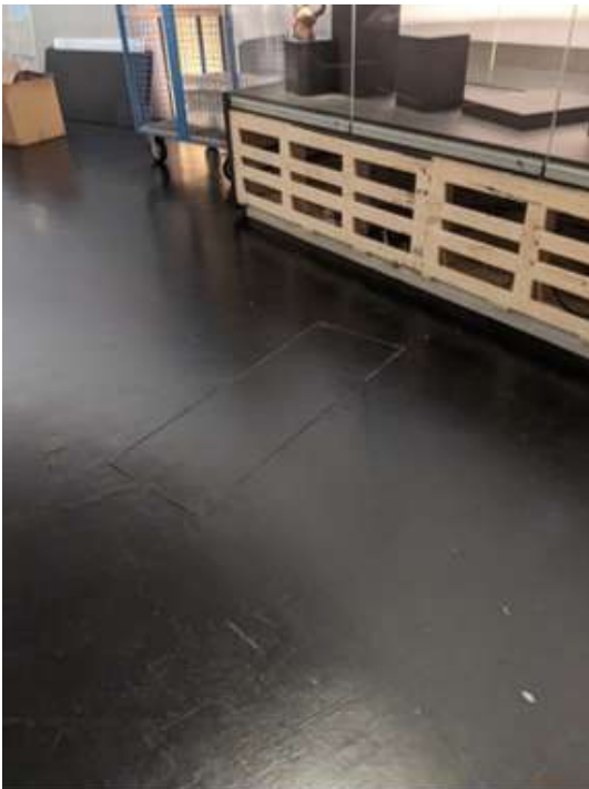
Above: existing ceiling, recessed lighting track and surface mounted fixtures to painted plasterboard ceiling. Left: existing cork floor tile finish, with inset floor box
