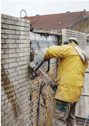
Cutting of external walls as panels
