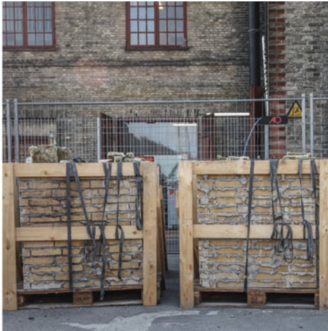
Cutting of external walls as panels
