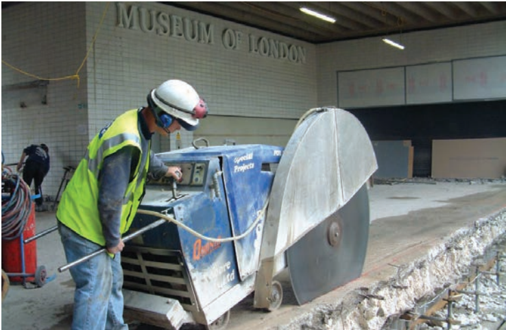
Diamond-saw cutting of RC slab as blocks
