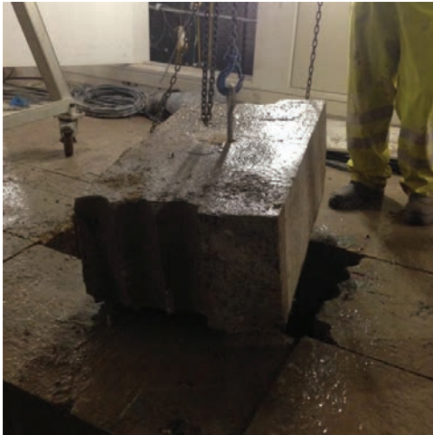
Diamond-saw cutting of RC slab as blocks
