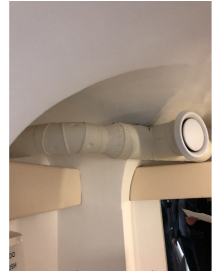
Existing toilet extract to be stripped out
