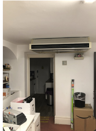
Existing ceiling mounted fan coil unit will be replaced
