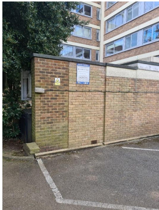
Rear of Site North- Possible Location 2
