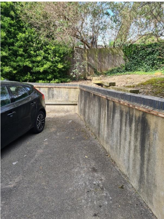
Rear of Site North- Possible Location 1
