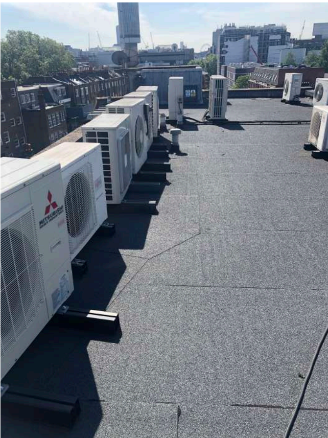
FIGURE 12. EXISTING ROOF-TOP PLANT - VIEWS ACROSS ROOF TO SOUTH
