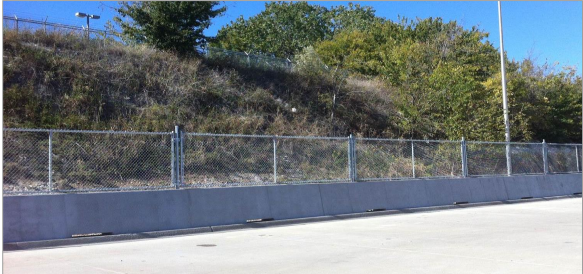
Figure 13 A Case study image of a metal chain link fence on top of a concrete upstand (this image is indicative only)
