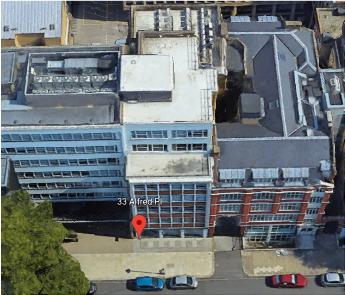
2. Front elevation and roof
