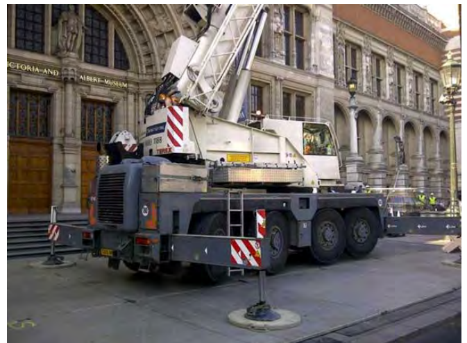
Crane positioned on riggers, transferring loading to the ground
