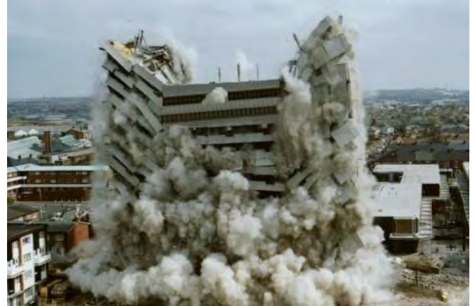
Demolition using explosives
