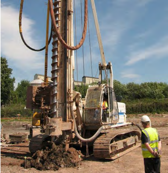
Continuous flight auger method of piling
