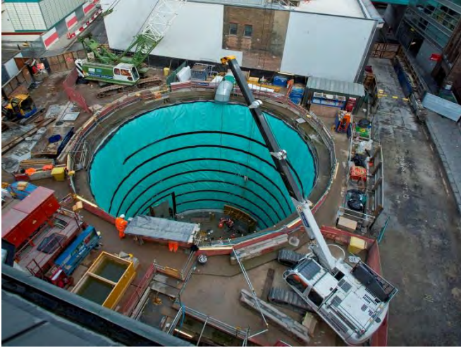
Deep excavation using heavy machinery
