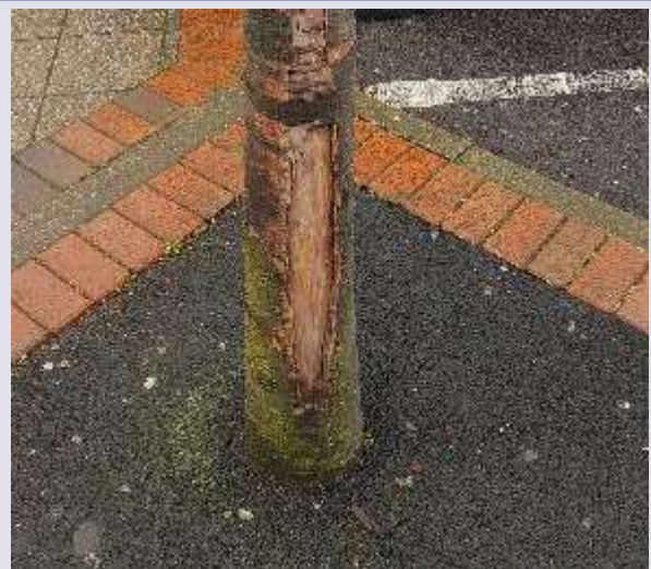
T022 with basal trunk damage. This type of damage is present on several trees.
