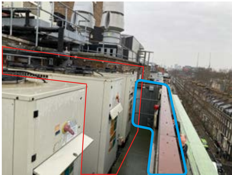
1. Existing chillers in acoustic enclosure to be replaced
