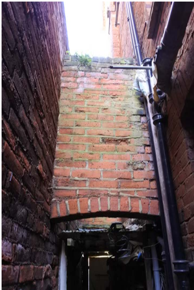
Photo of the brick structure that supports the side infill.
