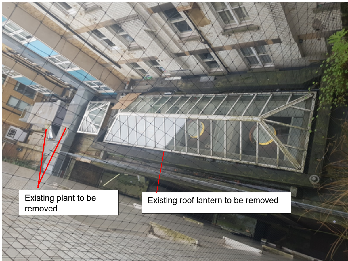
Figure 3: Photo showing existing roof lantern and plant to be removed
