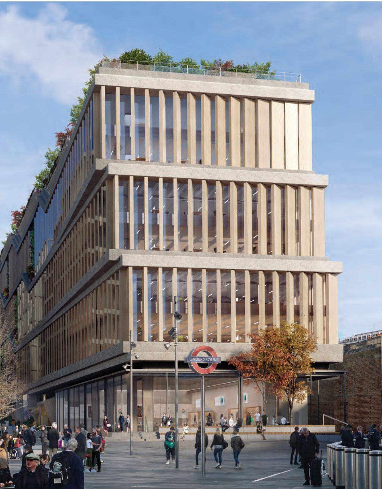
Figure 140: Illustrative view of the southern elevation of the building, showing the double height glazing and moving fins
