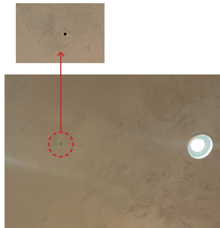
Example of installed aspirator smoke detection system, presents as small hole within ceiling systems
