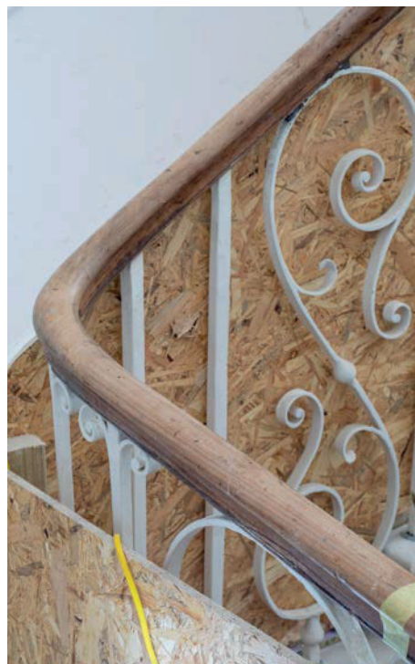
Main stair handrail to be refurbished
