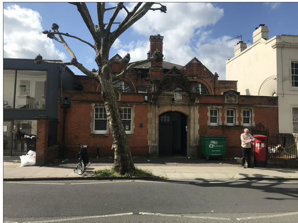
PHOTO OF EXISTING STREET ELEVATION
