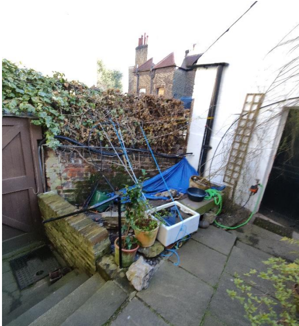
Photo from inside the courtyard of a makeshift attempt to prevent collapse (not sufficiently robust)
