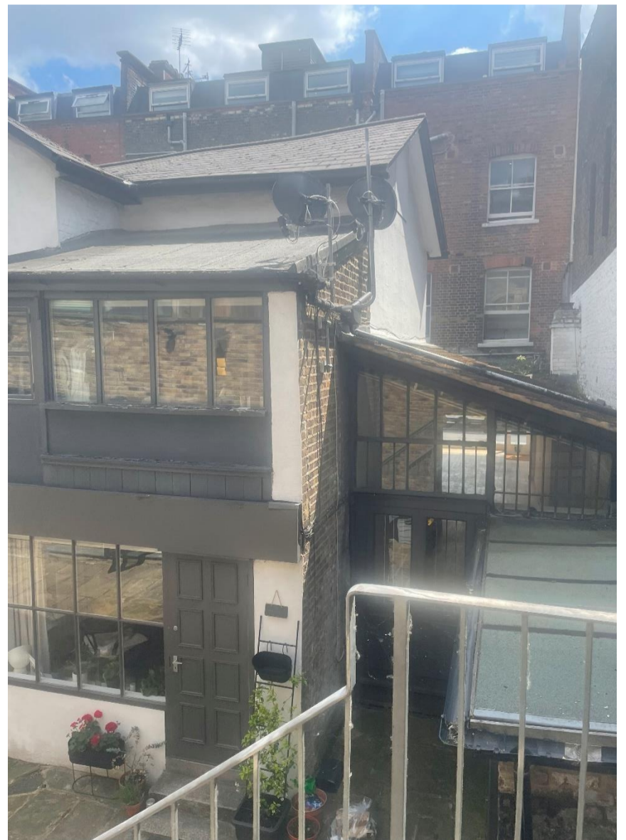
Looking on to rear elevation of Coach House (rear of street building) in residential use. Application site to left of page
